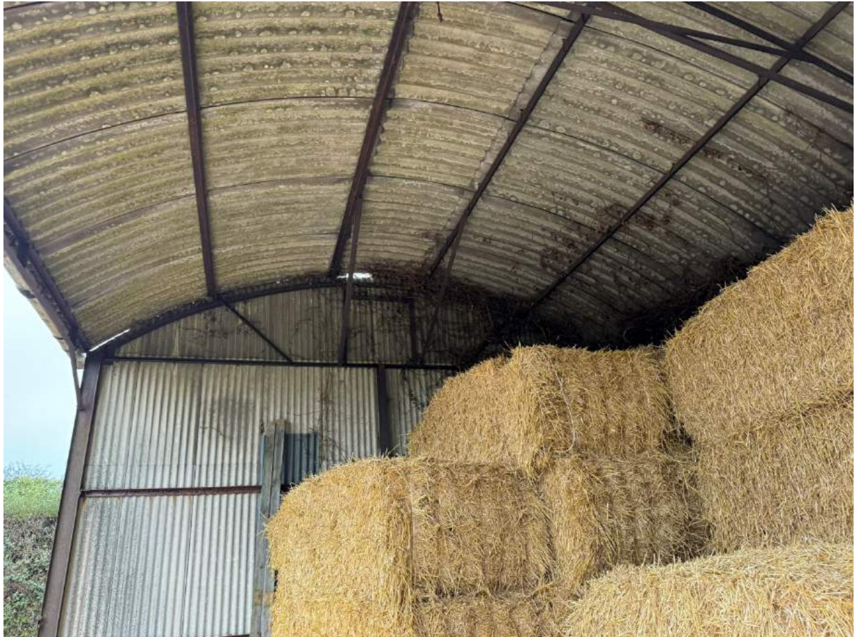
PHOTOGRAPH 5 – INTERNAL VIEW OF FRAME
