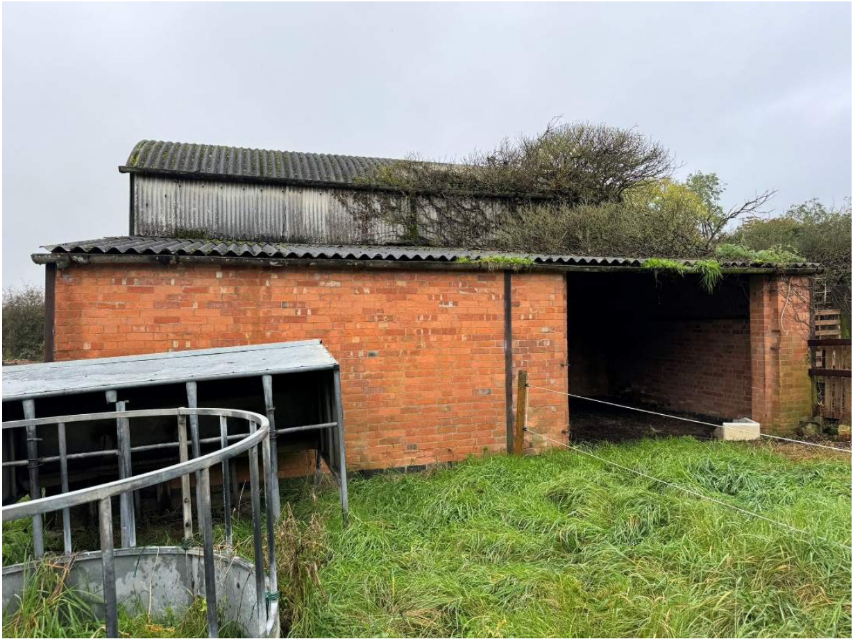
PHOTOGRAPH 4 –BARN REAR ELEVATION
