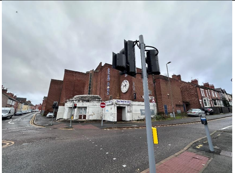
Image 1: Image looking at northern aspect of the building.
