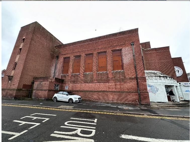
Image 4: Image looking at eastern aspect of the building.
