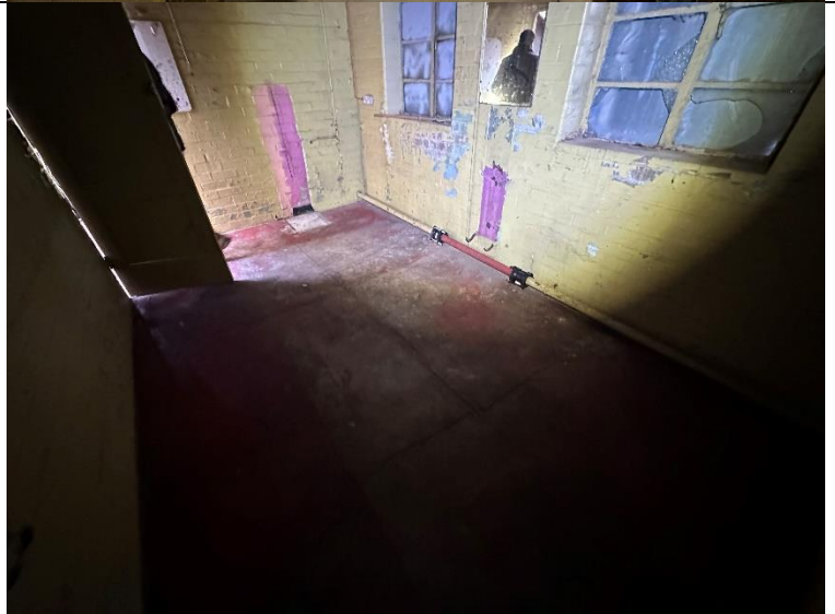
Image 17: Image showing internal condition of small room within the building.
