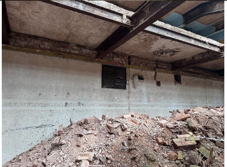
Image 14: Image showing internal condition of main section of the building.
