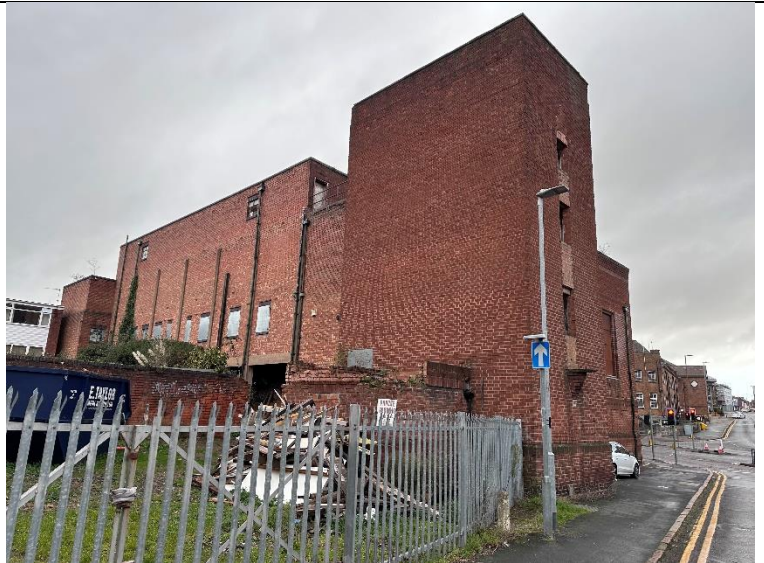
Image 5: Image looking at southern aspect of the building.
