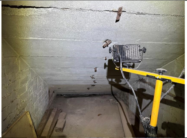
Image 16: Image showing internal condition of small room within the building.
