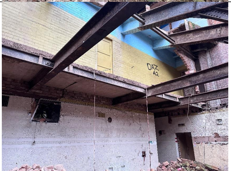
Image 15: Image showing internal condition of main section of the building.
