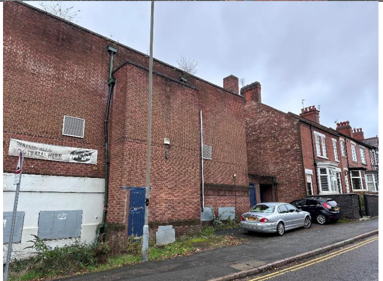
Image 2: Image looking at central section of the northern aspect of the building.
