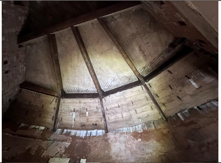
Image 13: Image showing roofed section of the entrance to the building.
