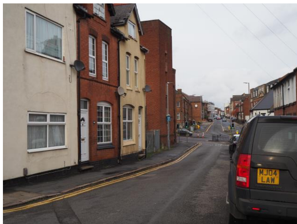
Fig 18: View along Trinity Lane towards Bond Street Circus with the lift / stair tower on the right side of the street
