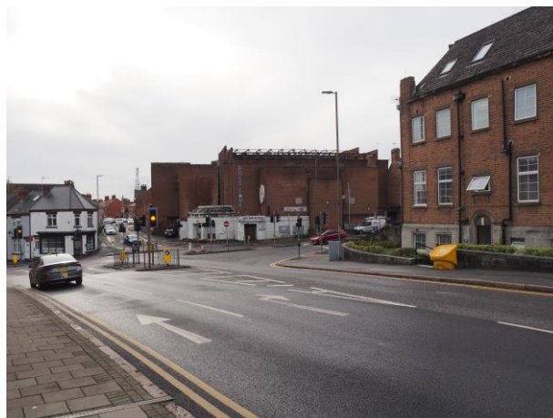
Fig 15: Former Danilo cinema from Upper Bond Street
