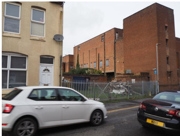
Fig 4: Side (south-west) elevation
