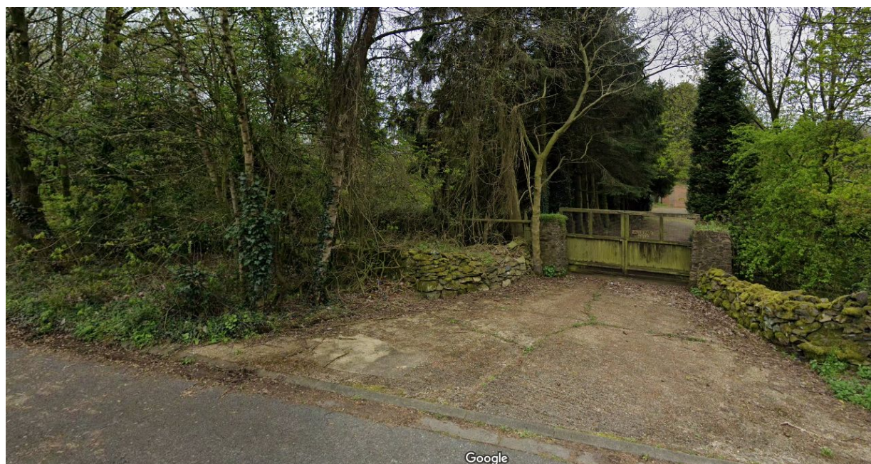
Image 5: Primary existing entrance from Altar Stones Lane
