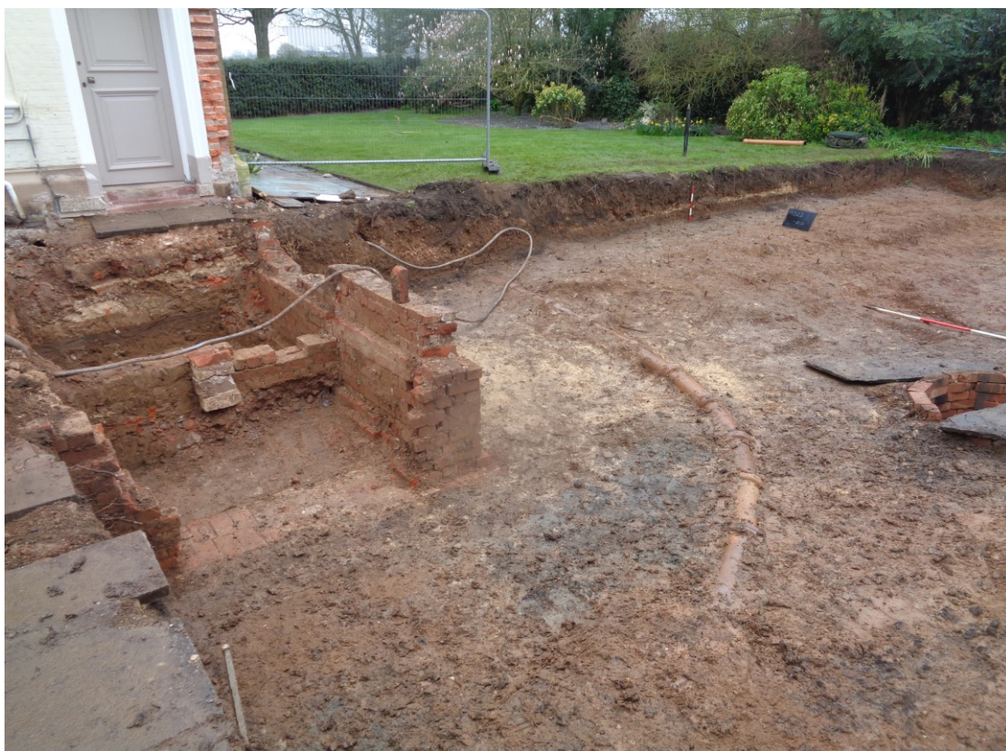
Plate 4: remains of former outbuildings, view southwest.
