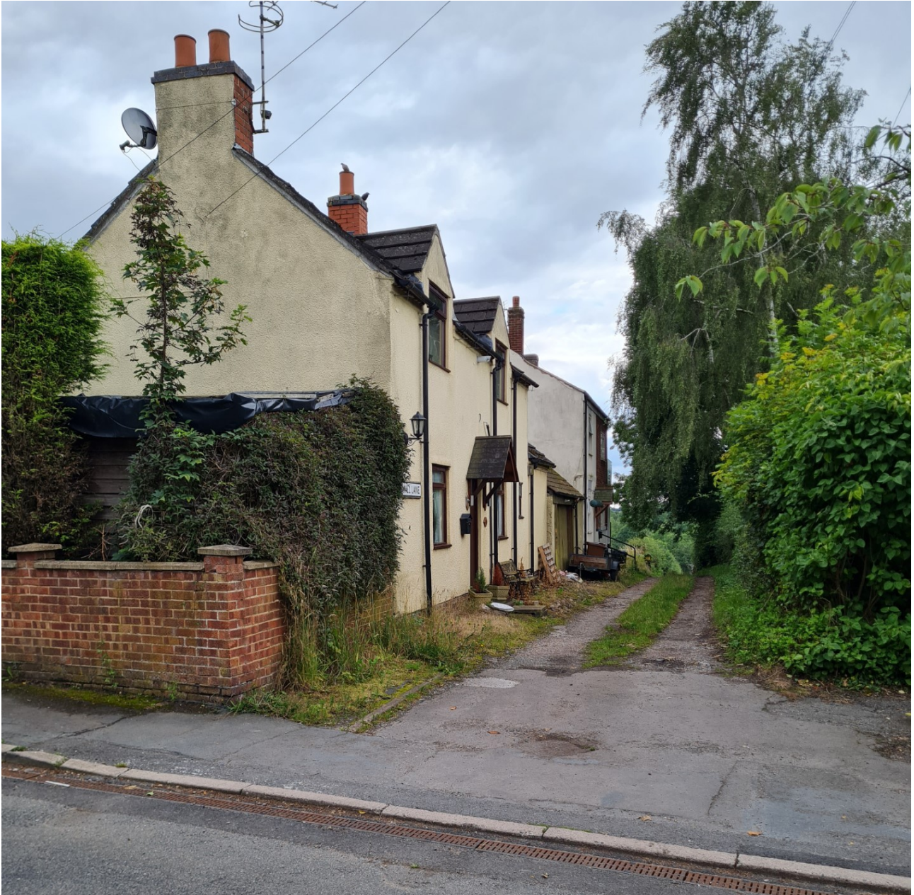
Figure 4 - View along Mill Lane from Main Street.
