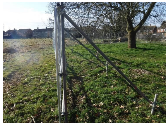
Photo 6: Scaffold driven into ground
