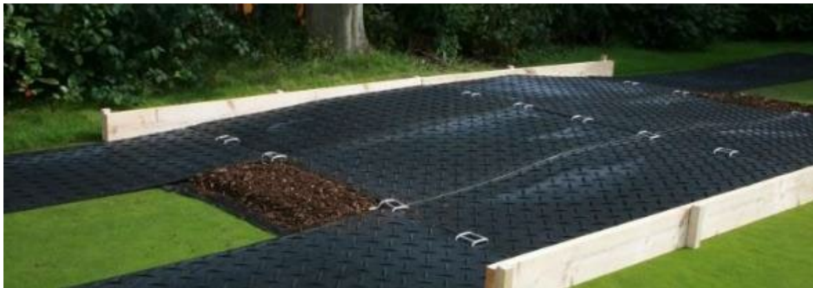
Image 1: Example of pedestrian operated machinery temporary ground protection
