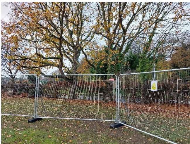
Photo 7: Heras fencing with base plate & sign. Strut (pinned)
