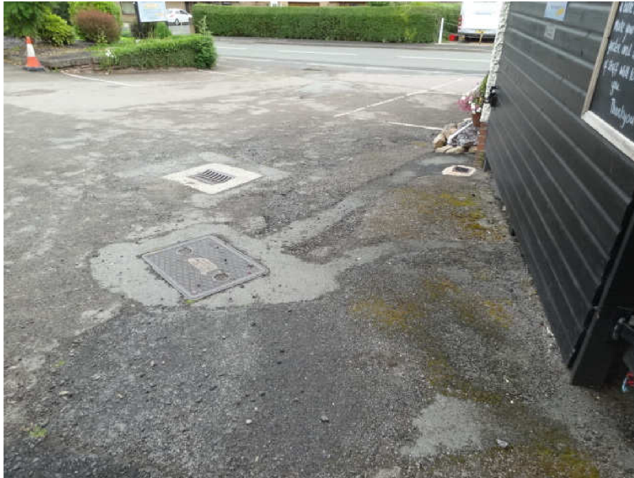
Photo showing tarmac car park area; J5
