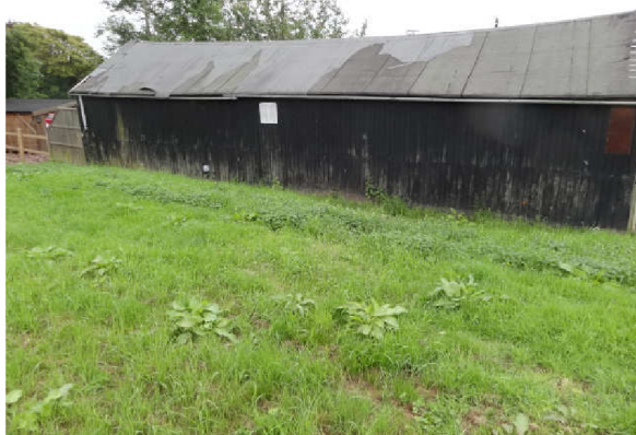
Photo showing rear of function room
