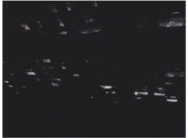
Church Cottage roof void showing gaps between tiles
