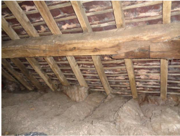
Church Cottage roof void
