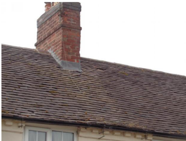
Northern aspect of roof
