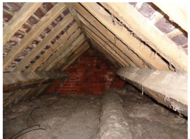
Church Cottage roof void
