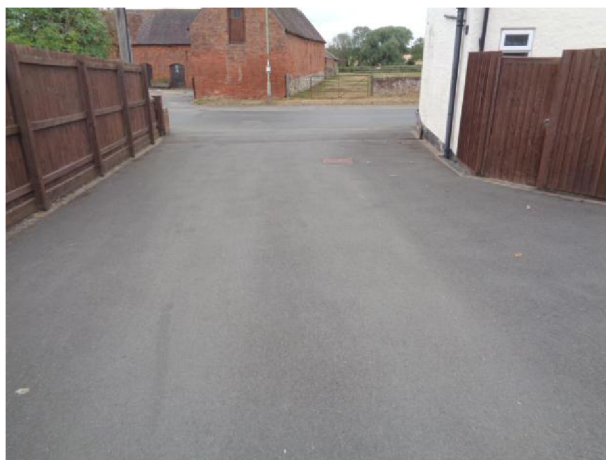
Boundary across hardstanding
