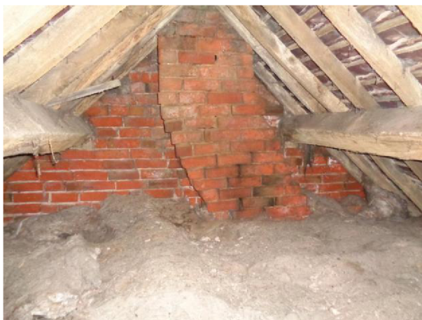
Church Cottage roof void
