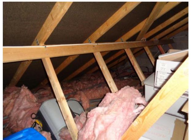
Roof void of offices
