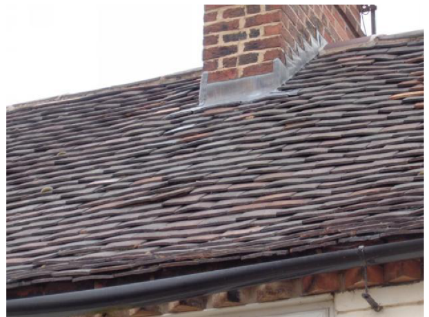
Southern aspect of roof
