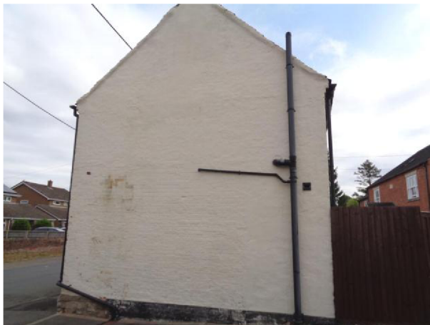
Church Cottage western aspect
