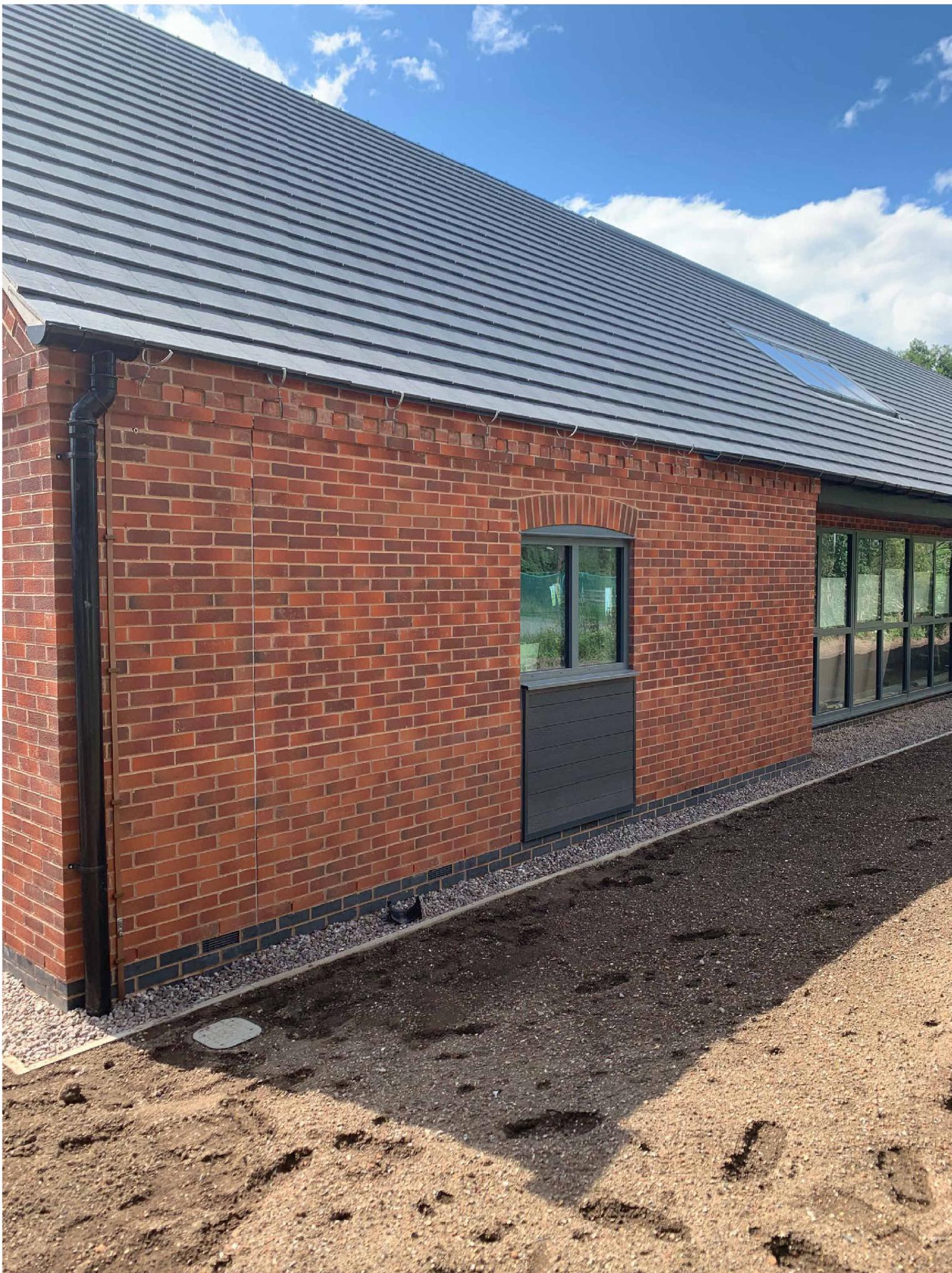
Existing External View
