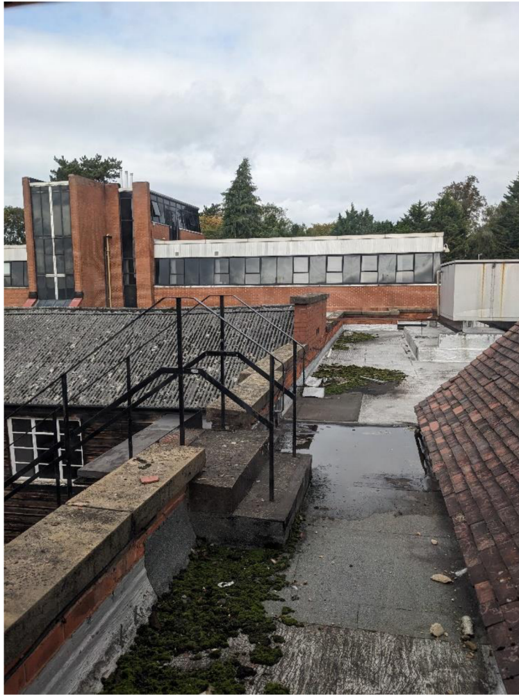
Plate 7 – Rooftop of main building.
