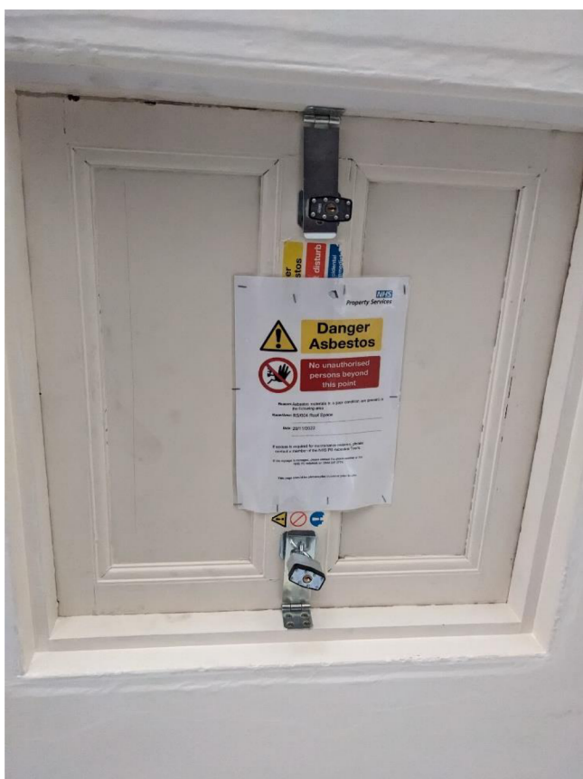
Plate 14 – Loft closed due to asbestos risk.
