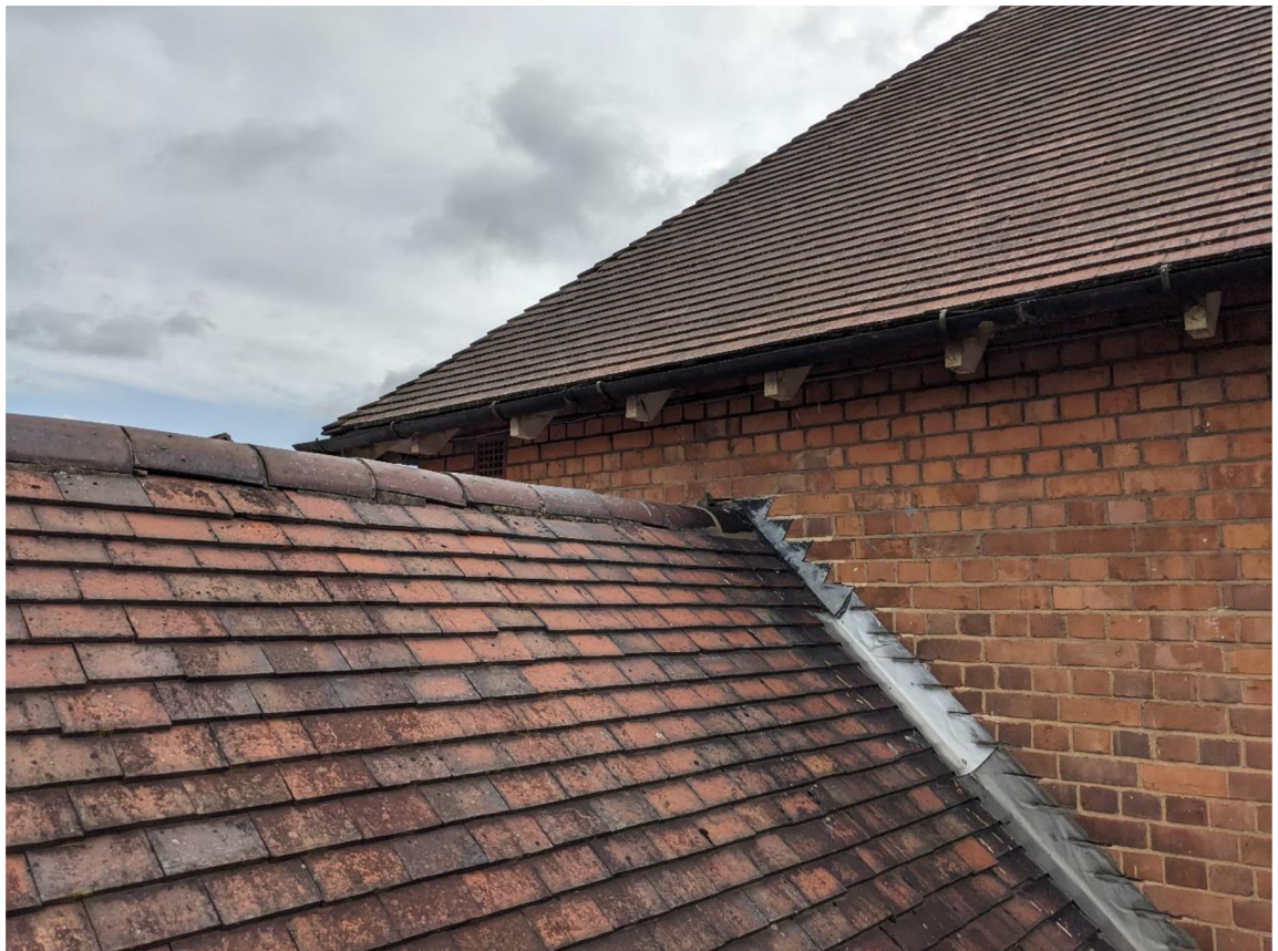
Plate 8 – Close up of eaves and ridge tiles.
