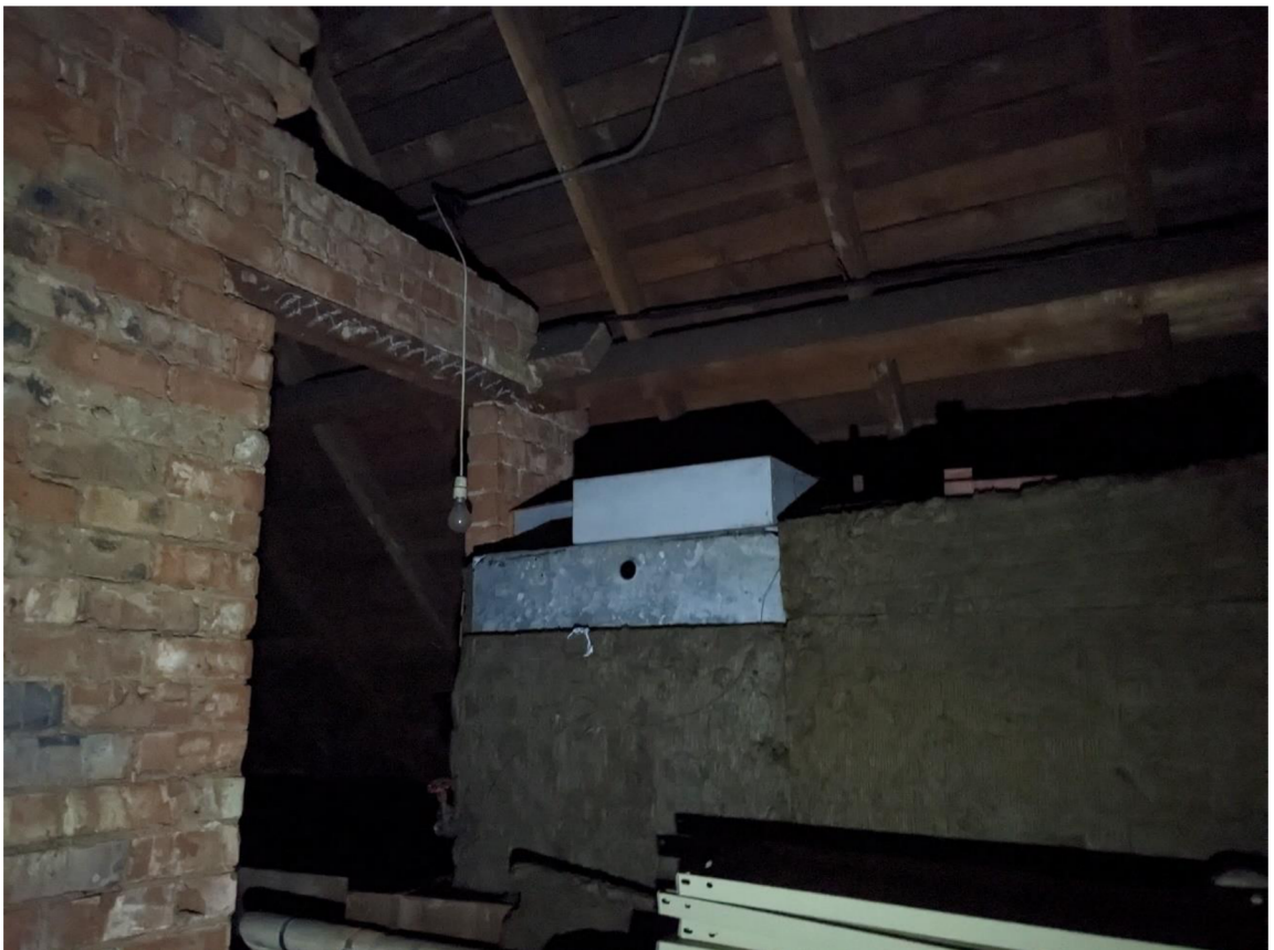
Plate 18 – Ceiling of the main internal loft space.
