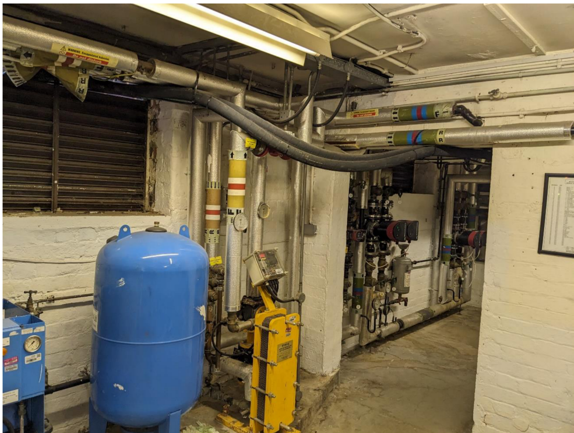
Plate 11 – Internals of basement areas.
