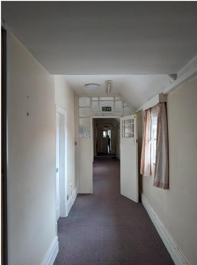
Plate 15 – Example of internal corridor showing lack of loft space for the majority of the building.
