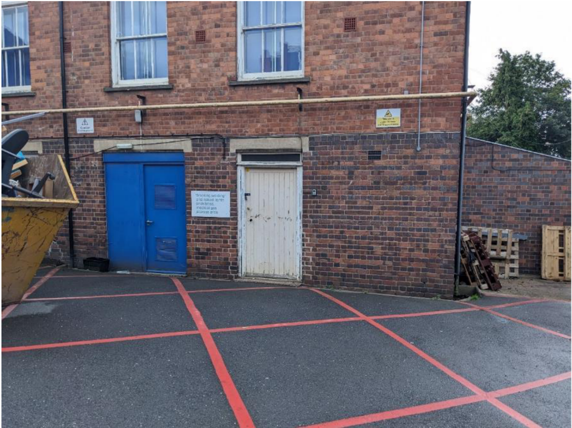
Plate 1 – General view of the northern aspect.
