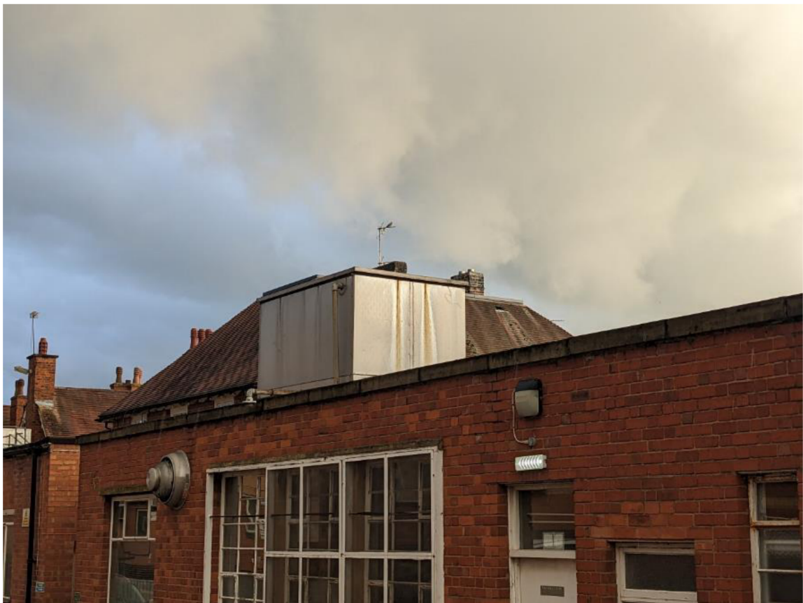
Plate 4 – eastern aspect roof.
