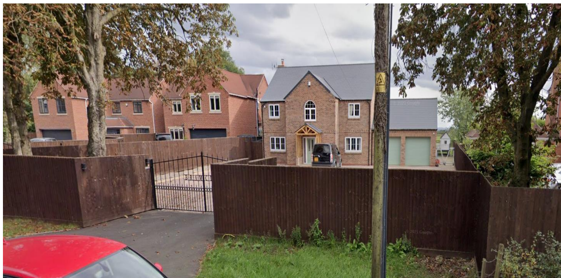
Photograph 8 –new housing – further south along Thornton Lane
