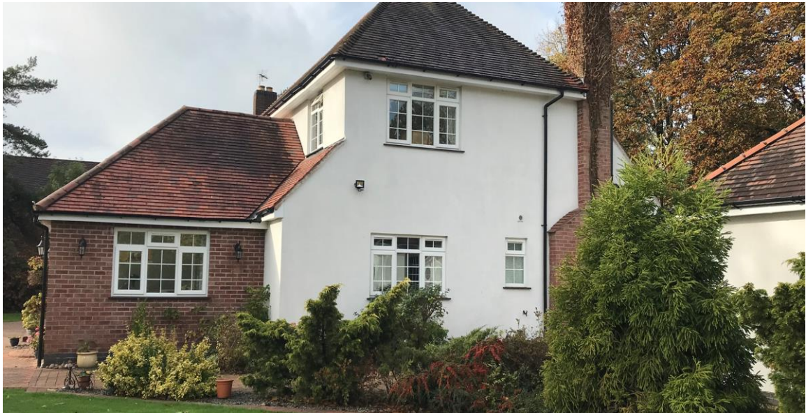
Photograph 6 – facing elevation of Ben Venuto (containing dining room, bedroom and WC windows)
