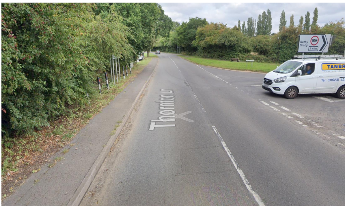
Junction with Ratby Lane – level footway with benches and communal areas
