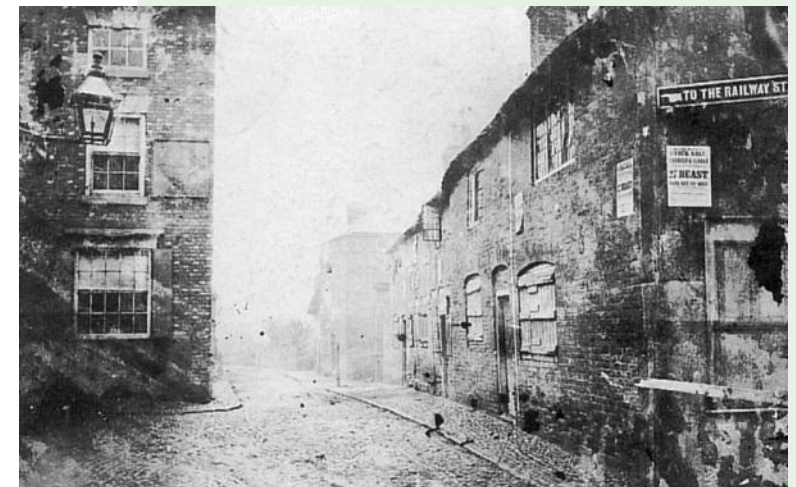
Station Road before demolition
