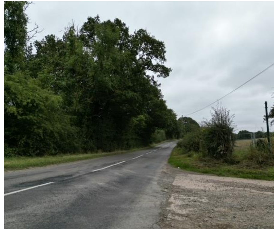
Figure 4. Facing south on Markfield Road.
