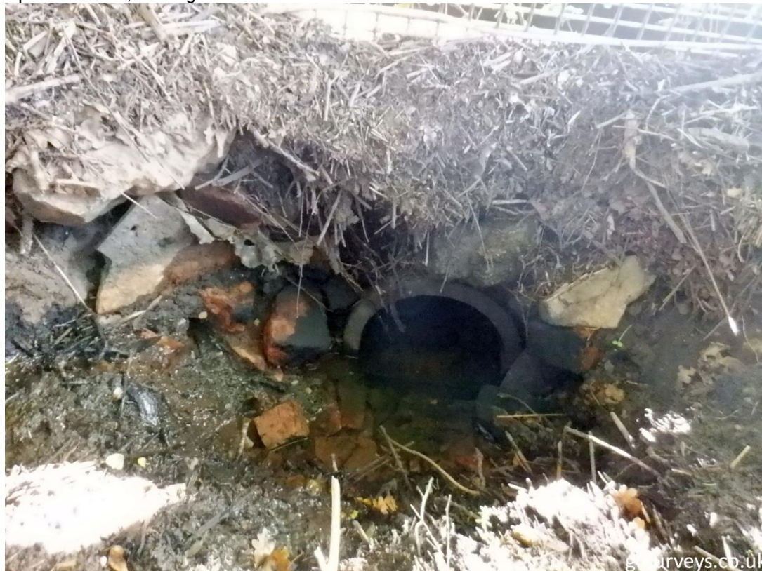
Upstream face, looking downstream
