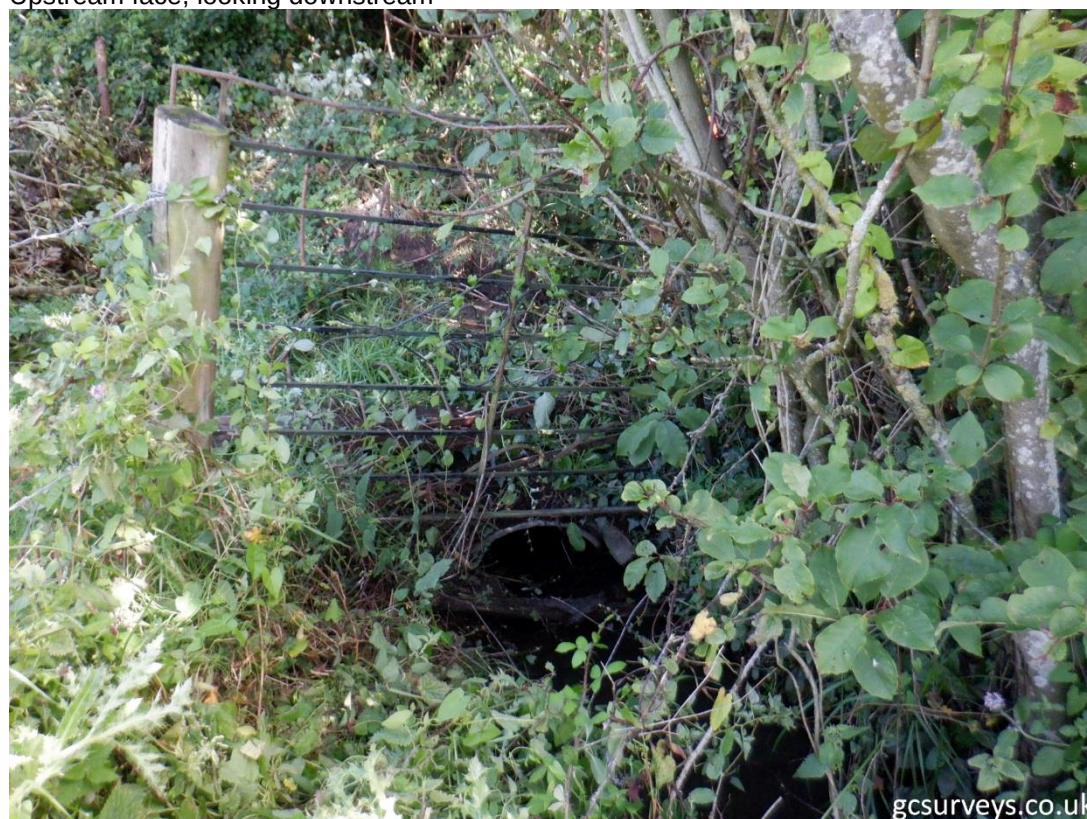
Upstream face, looking downstream
