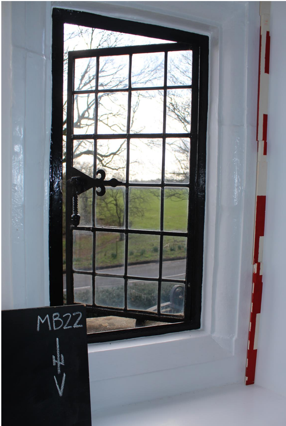
Plate 9: Detail of window's iron fittings and furnishings.
