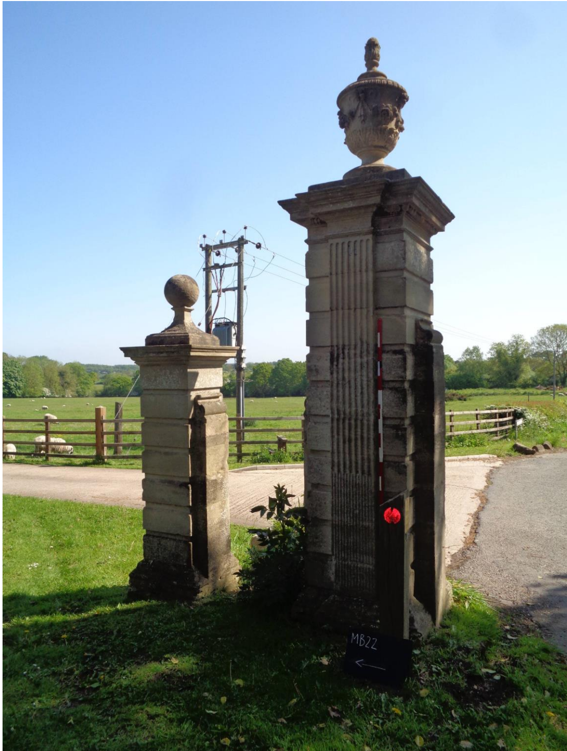
Plate 26: The northern gate-piers, from southwest.
