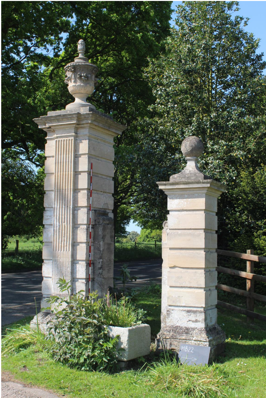
Plate 25: The northern gate-piers, from northeast.
