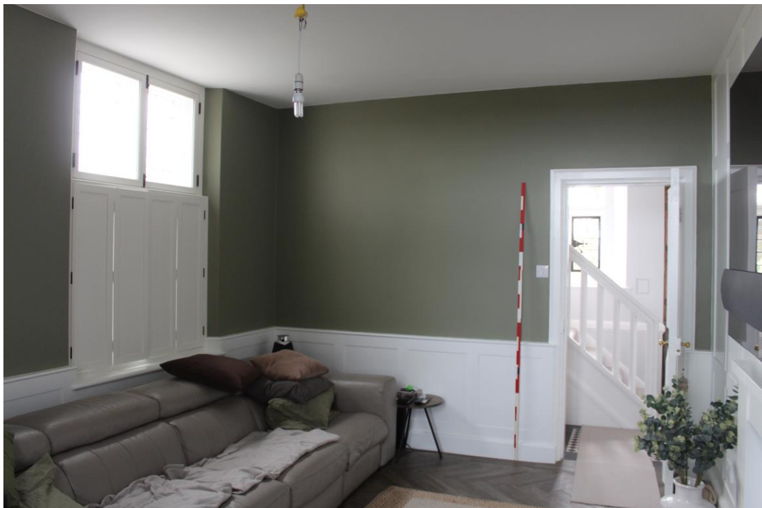
Plate 14: The former parlour, the dado-panelling and window shutters are modern features, and the fireplace which replaced the original, on the right, has been panelled over.
