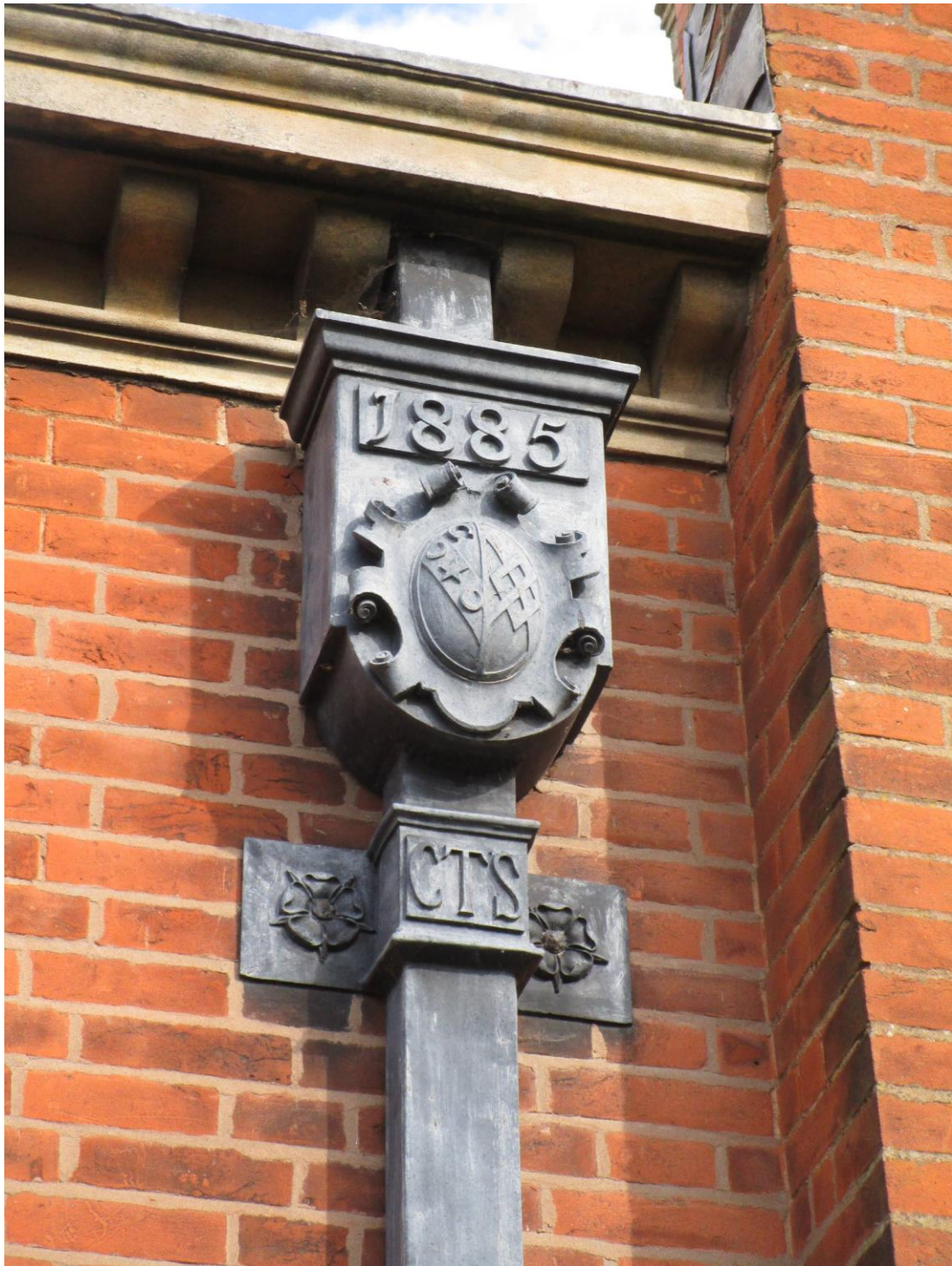
Plate 6: View of hopper and rainwater pipe detail.
