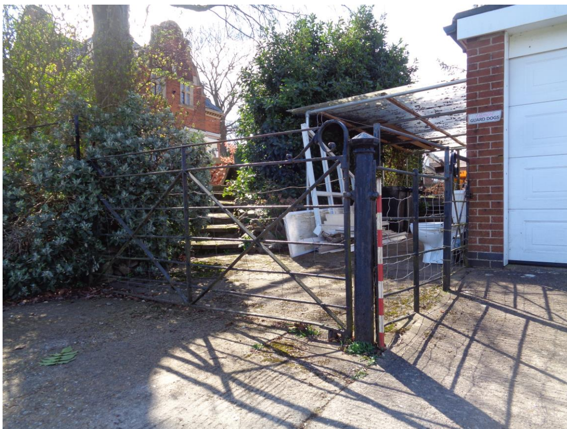
Plate 21: View of rear gates from northeast.
