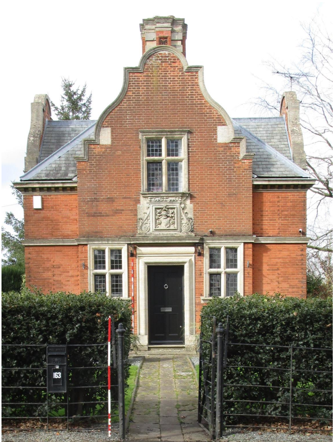
Plate 7: View of front gate from south.
