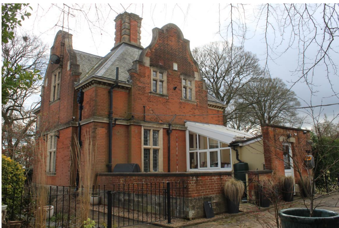
Plate 3: View from northeast, note the repaired brickwork following the removal of kitchen-yard wall around northeast corner. The rendered wall is the surviving west wall of the coal-shed.
