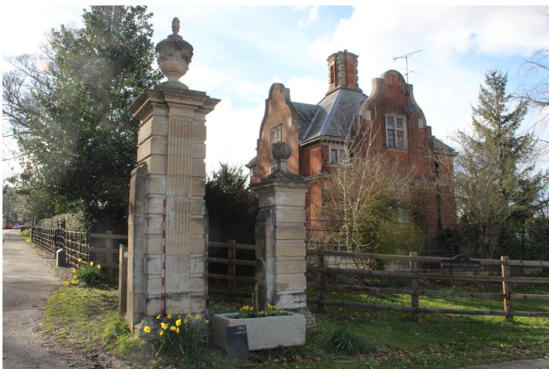
Plate 5: View of northern gate piers and the lodge beyond, from southeast.
