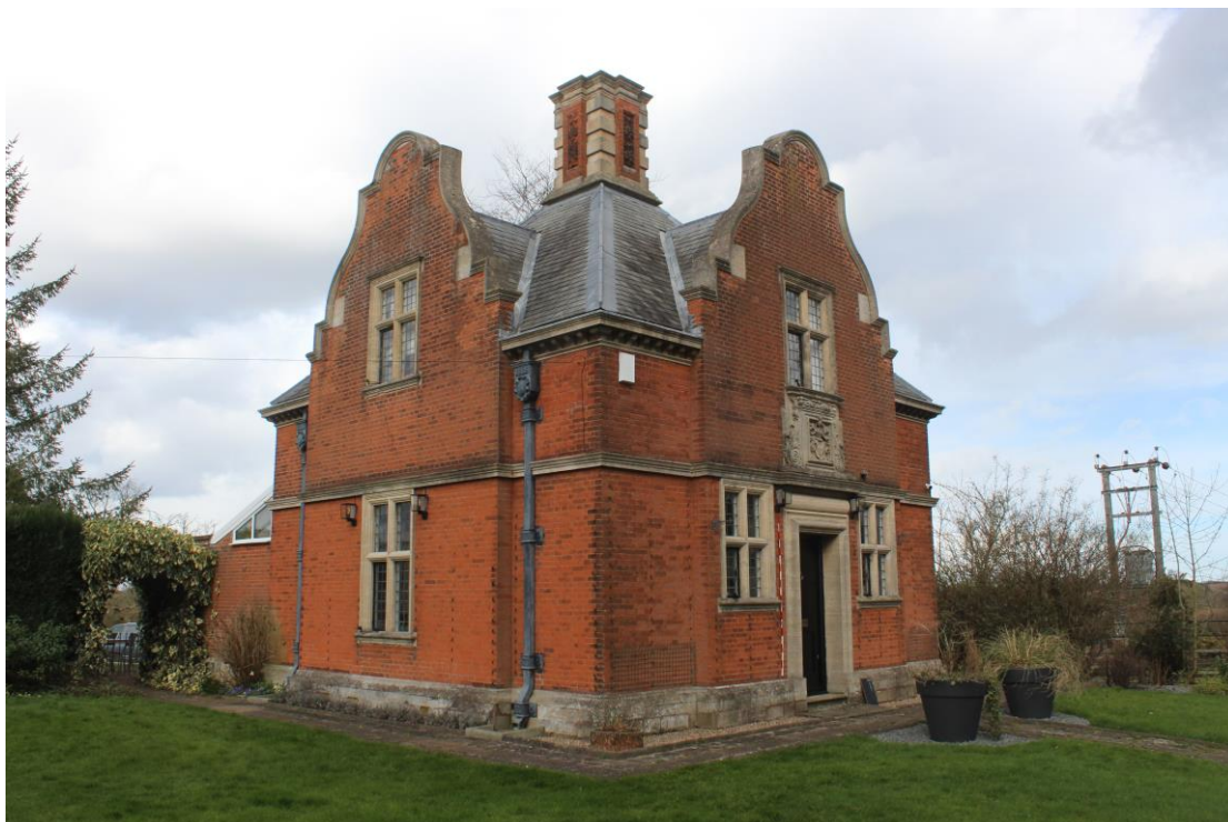
Plate 2: View from southwest.
