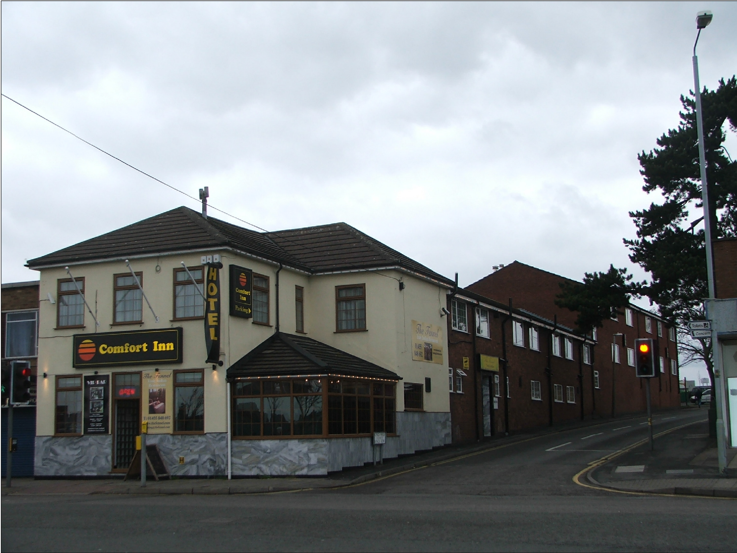
PHOTO AS EXISTSING
