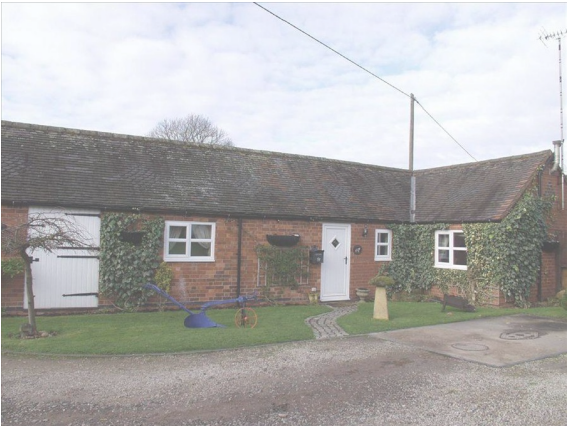
Photo of Existing Front Elevation
