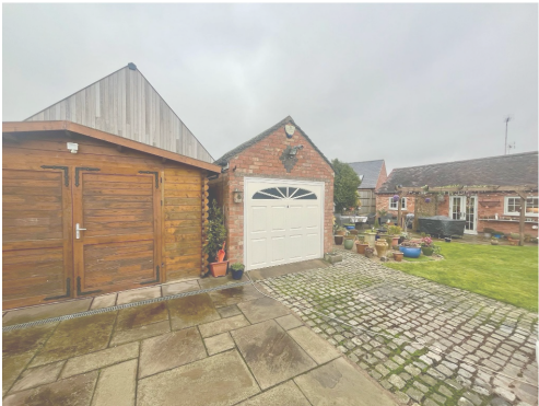
Existing rear garden & outbuildings buildings
