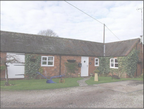
Photo of Existing Front Elevation
