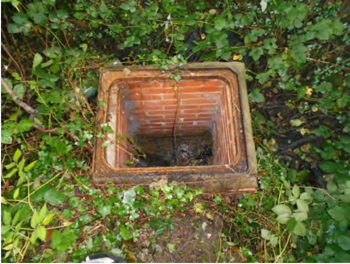
LOCATION REAR OF FOOTPATH ON OLD A47
