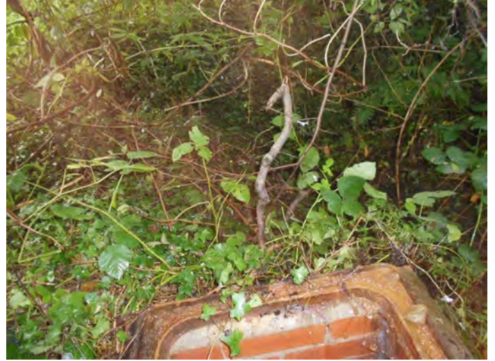
HIGHWAY DITCH INCOMING
