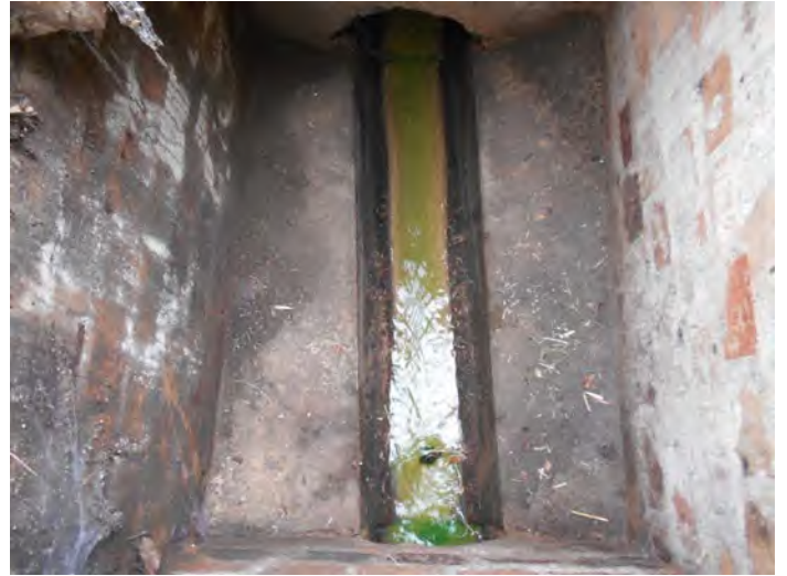
DYE TEST FROM IFHW1 IN CHAMBER TO PROVE CONNECTION
