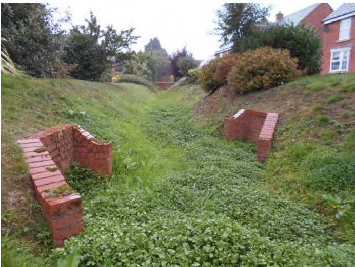
OPEN DRAINAGE DITCH LOOKING TOWARDS GARNER CLOSE
