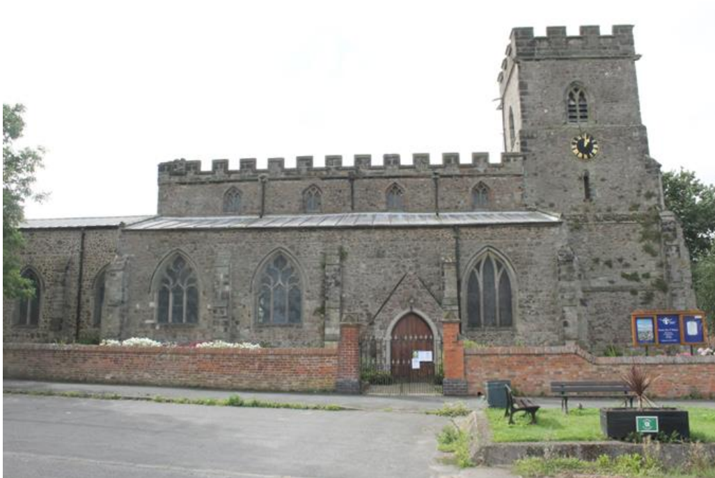
Plate 1 Church of St Mary, Barwell (1074669)
