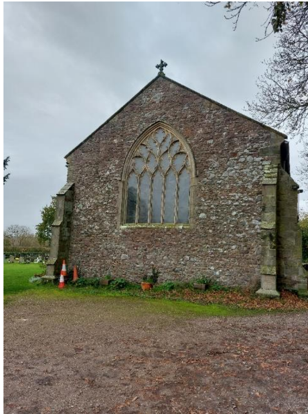
Plate 12 Rear of St Mary's Church Elvesthorpe (1074693)
