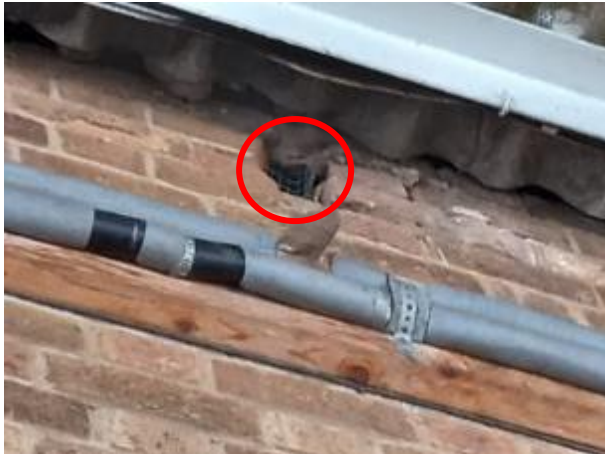
Plate 3.18: Possible gap between mesh and brickwork that may provide bats with access into the original building
