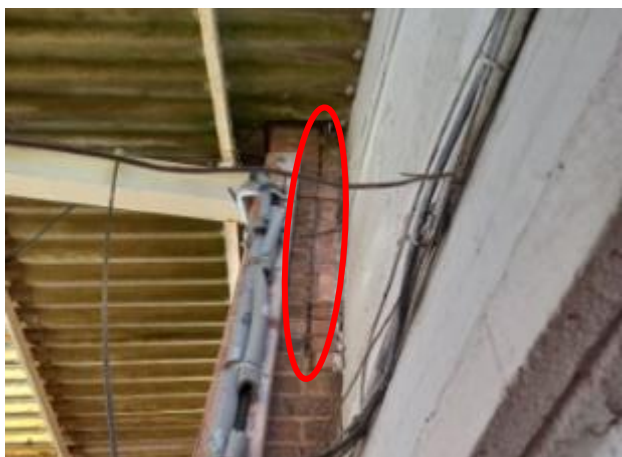
Plate 3.17: Possible crevice in between the two skins of the wall at the northern end of the parapet wall
