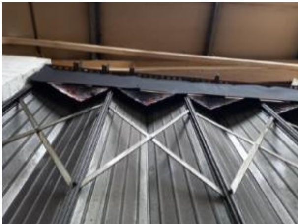
Plate 3.23: Daylight visible at top of folding doors
