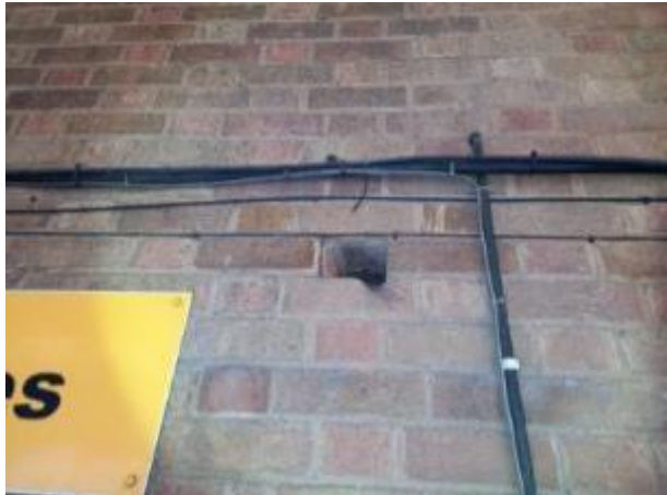
Plate 3.19: Hole into wall on eastern elevation of original section
