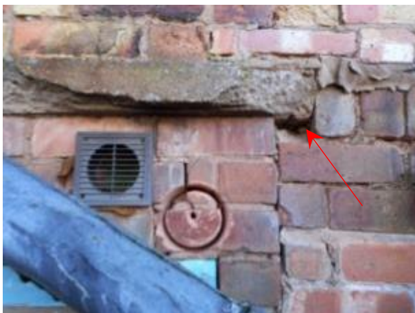
Plate 3.16: Missing mortar on northern elevation (main section) that leads into a small crevice in the wall (indicated with arrow)
