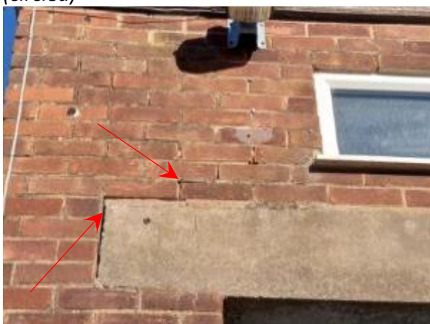
Plate 3.22: Gap around lintel on main extension, leading to shallow crack in brickwork (indicated with arrows)
