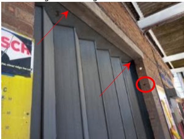
Plate 3.20: Gaps at top of folding doors and between lintel and door frame (indicated by arrows), and where rotten wood has created gap into a small cavity between brick skins (circled)
