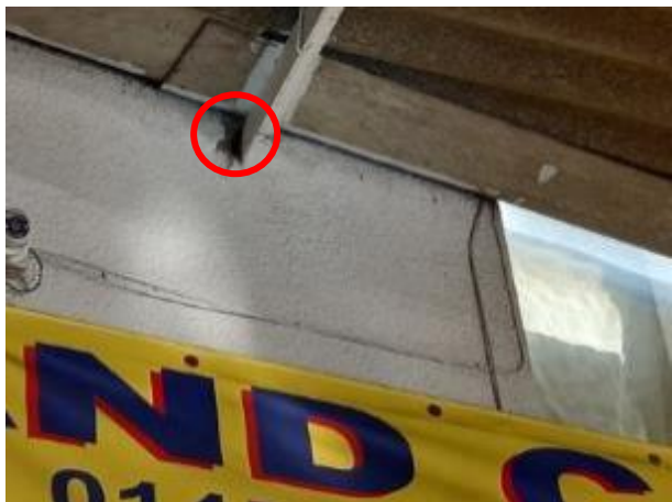
Plate 3.21: Example of gap between canopy beam and the brickwork of the adjoining house
