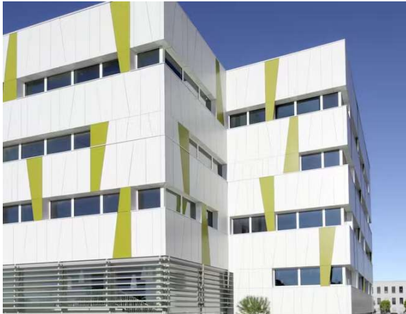
Figure 3 - Rockpanel Cladding shown in situ.
