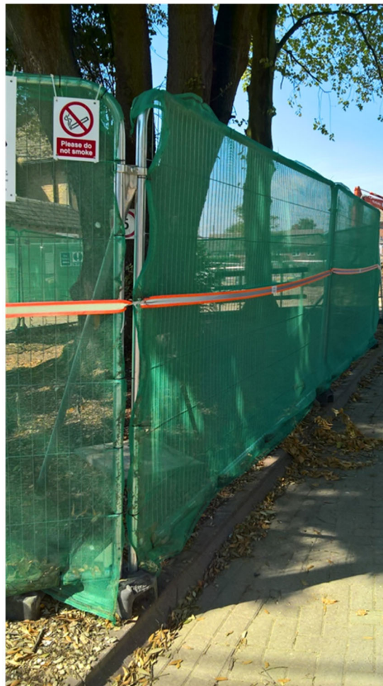
Photograph 4 (Example of tree protection barriers placed adjacent to existing hard surface &/or temporary ground cover)
