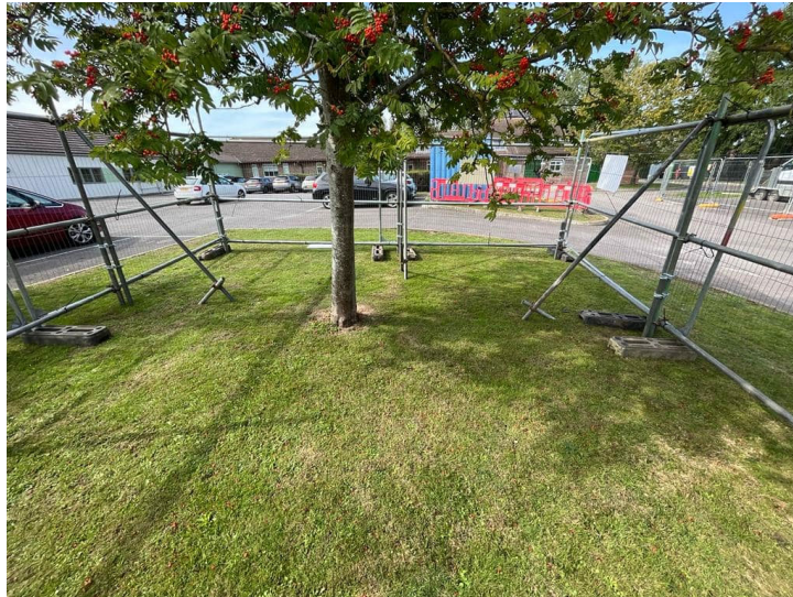
Photograph 3 (Onsite example of tree protection barriers)
