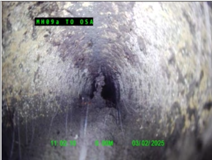
Start node type, Manhole, reference MH09a
