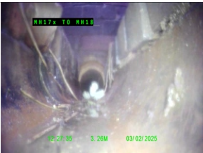
Finish node type, manhole, reference MH18
