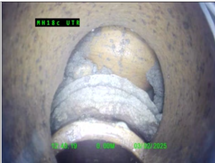
Start node type, Manhole, reference MH18c
