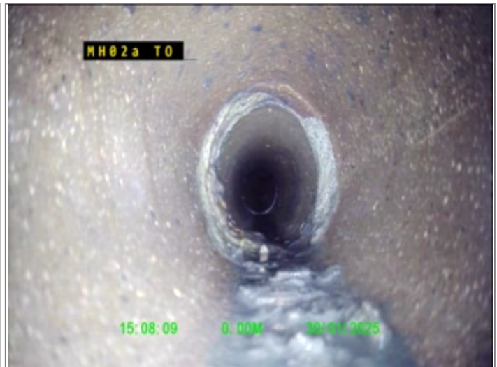
Start node type, Manhole, reference MH02a
