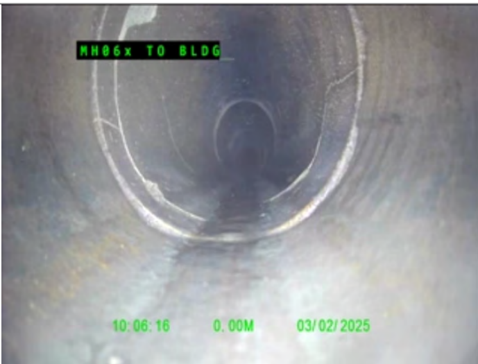
Start node type, Manhole, reference MH06x
