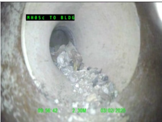
Loss of vision, silt, Finished
