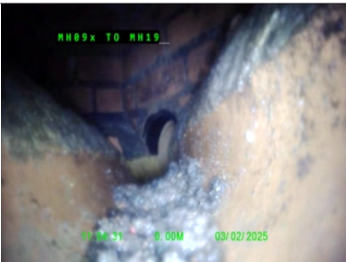
Finish node type, manhole, reference MH19
