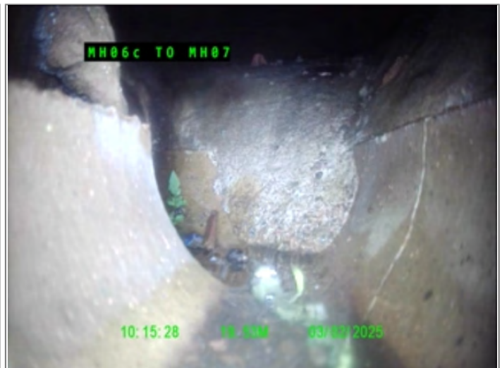
Finish node type, manhole, reference MH07
