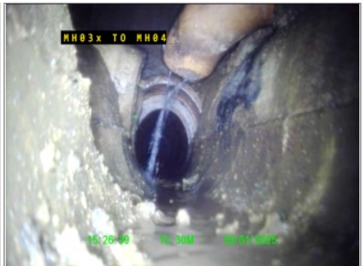
Finish node type, manhole, reference MH04
