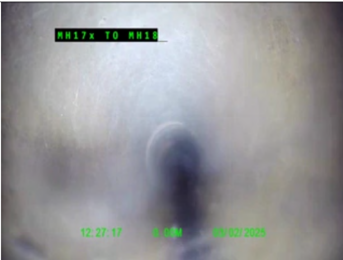
Start node type, Manhole, reference MH17x
