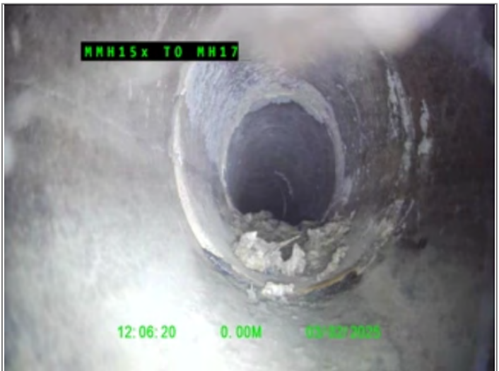
Start node type, Manhole, reference MH15x
