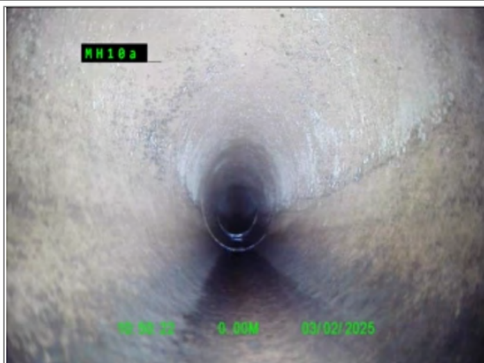
Start node type, Manhole, reference MH10a
