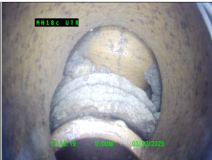
Collapsed drain/sewer 70%
