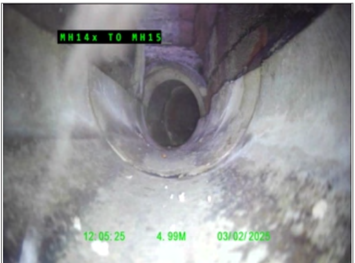
Finish node type, manhole, reference MH15
