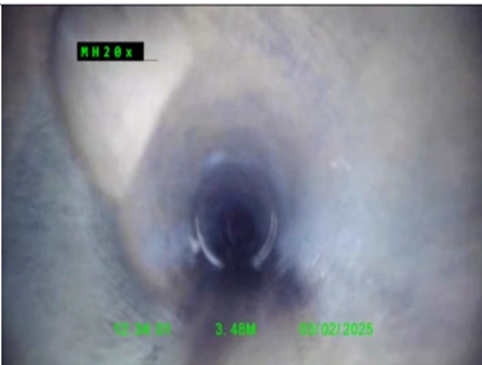
Connection other than junction at 10 o'clock, diameter 100mm
