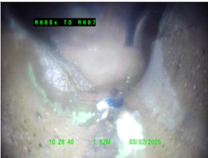
Finish node type, manhole, reference MH07
