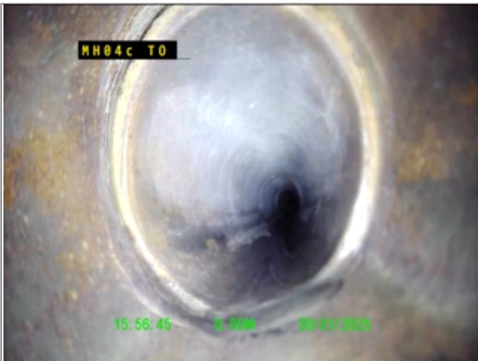
Start node type, Manhole, reference MH04c
