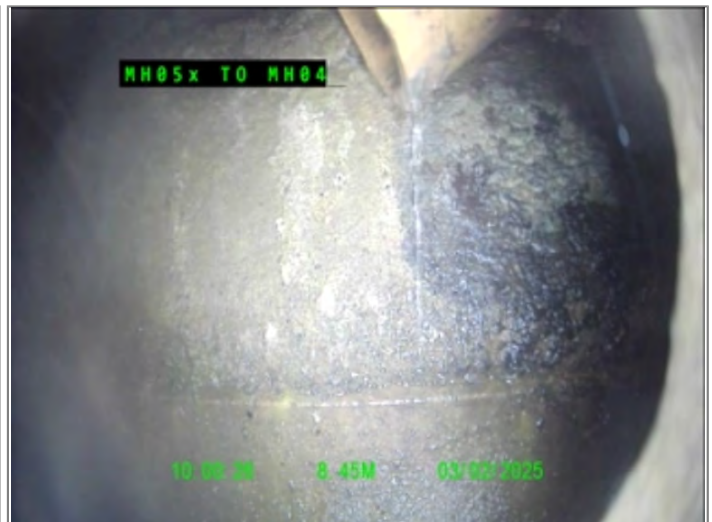
Finish node type, manhole, reference MH04
