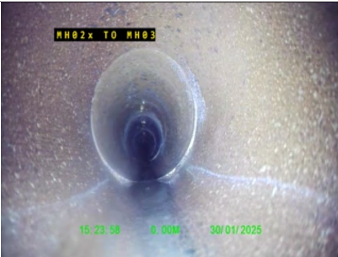
Start node type, Manhole, reference MH02x
