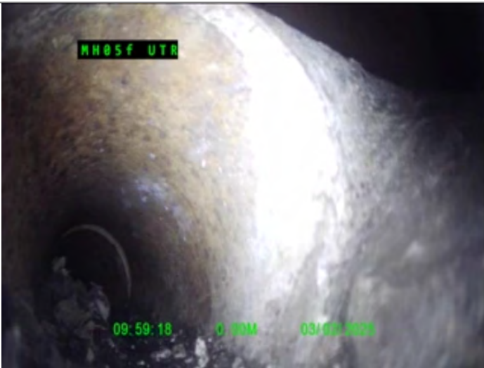
Start node type, Manhole, reference MH05f
