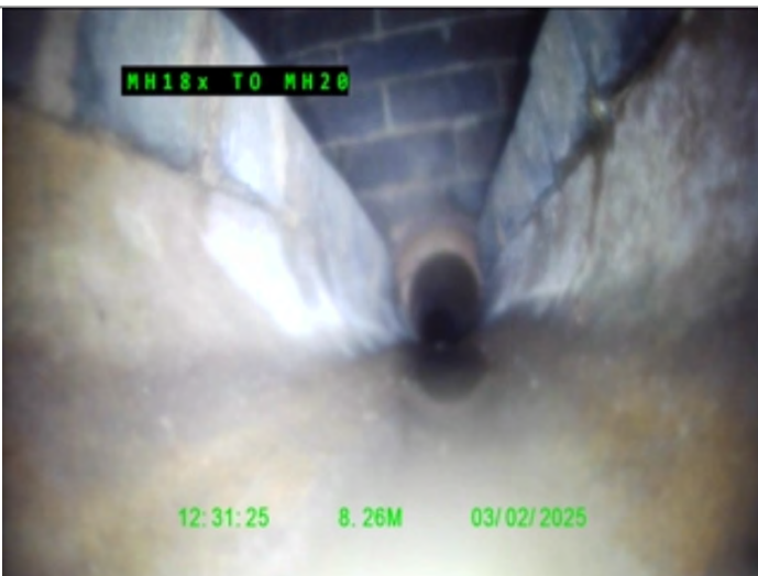
Finish node type, manhole, reference MH20
