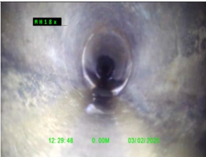
Start node type, Manhole, reference MH18x
