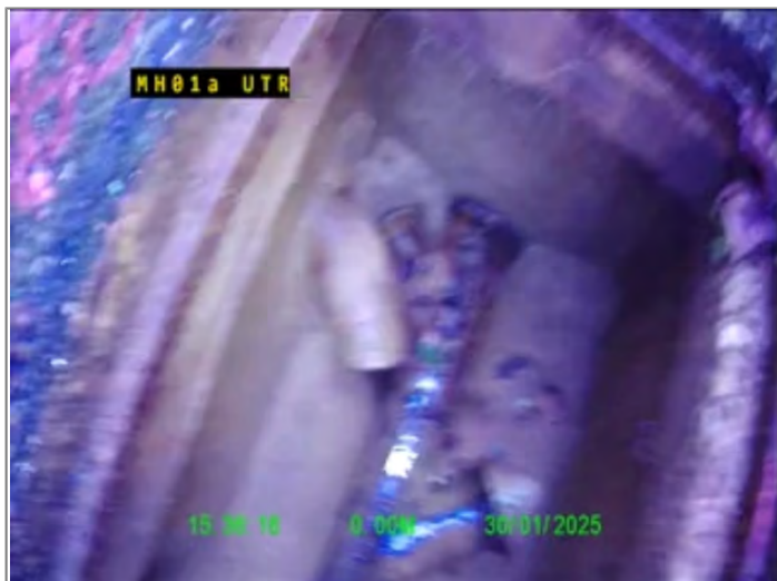
Start node type, Manhole, reference MH01a
