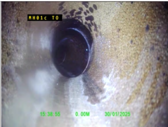
Start node type, Manhole, reference MH01c
