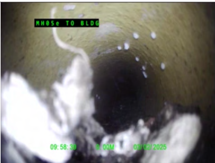
Settled deposits hard or compacted 40% cross-sectional area loss, Start
