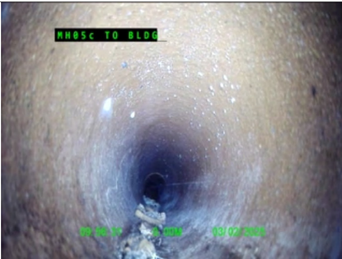
Start node type, Manhole, reference MH05c
