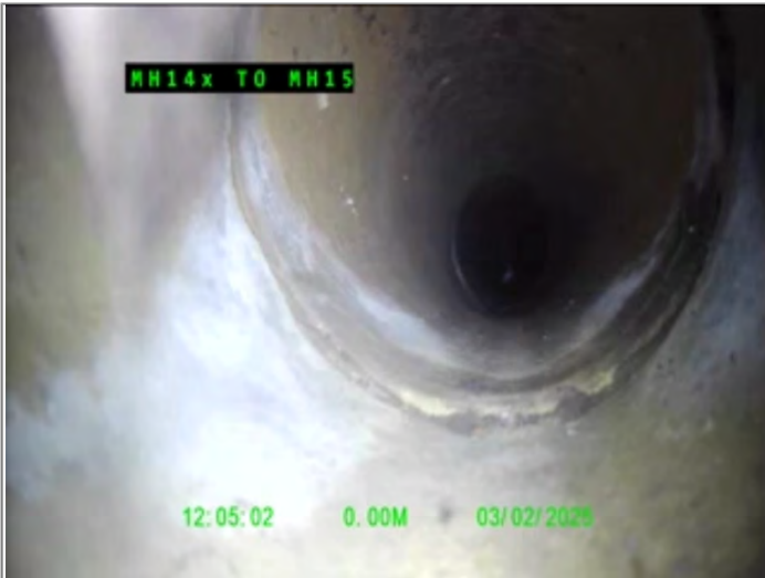
Start node type, Manhole, reference MH14x
