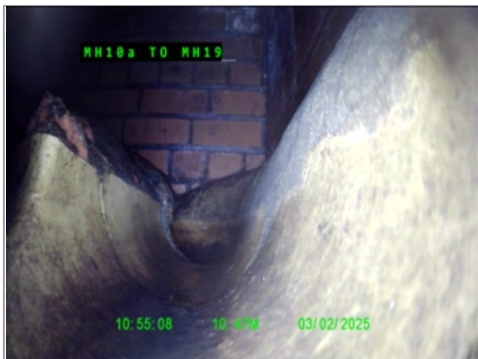
Finish node type, manhole, reference MH19
