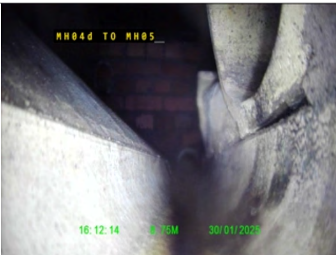
Finish node type, manhole, reference MH05
