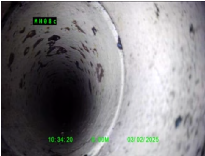
Start node type, Manhole, reference MH08c
