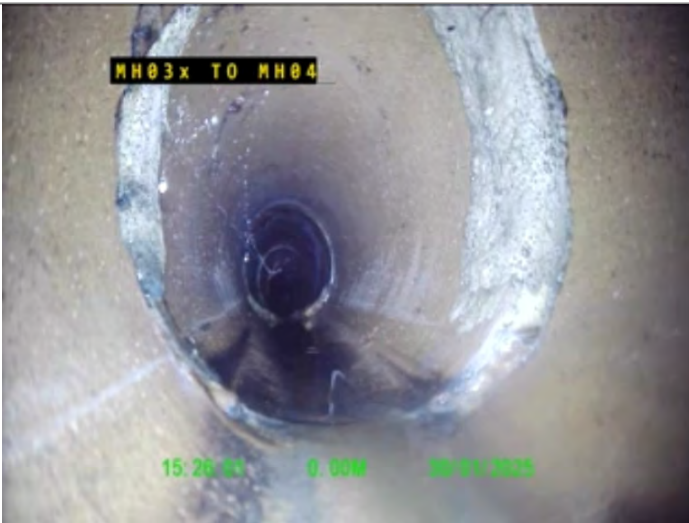
Start node type, Manhole, reference MH03x
