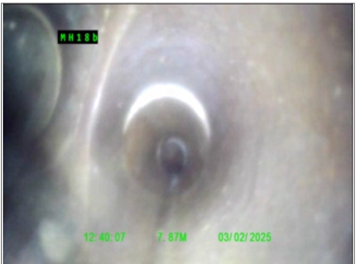
Connection other than junction, closed, at 9 o'clock, diameter 100mm
