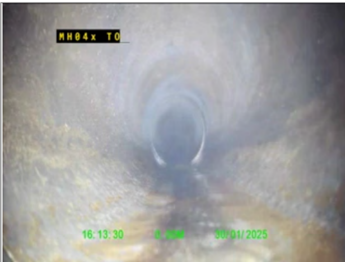
Start node type, Manhole, reference MH04x
