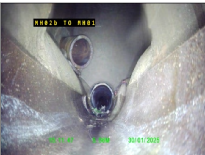
Finish node type, manhole, reference MH01
