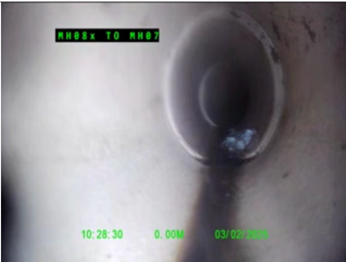
Start node type, Manhole, reference MH08x
