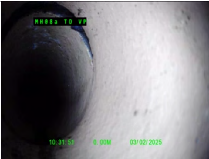
Start node type, Manhole, reference MH08a
