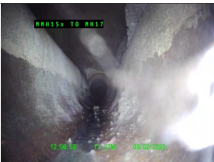
Finish node type, manhole, reference MH17
