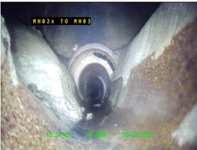
Finish node type, manhole, reference MH03
