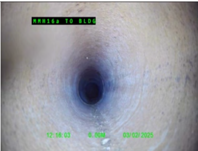
Start node type, Manhole, reference MH16a
