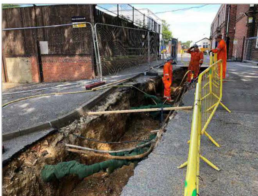
Figure 5 – Retained roots in service trench
