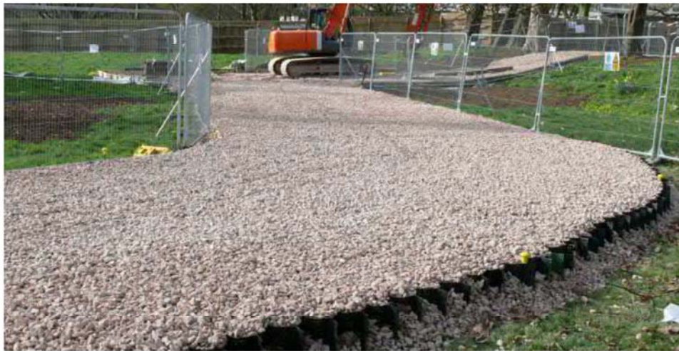
Figure 4 - Example of temporary Cellweb® construction solution
