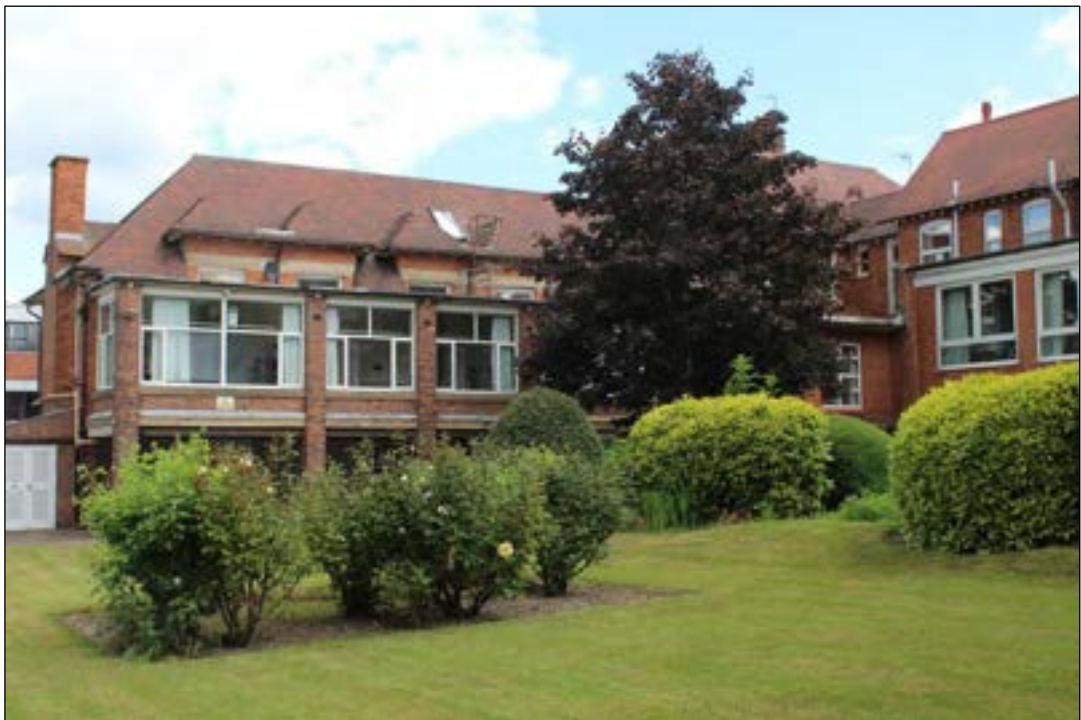
Photo 8 North part of the west-facing elevation of the 1938 extension to the Cottage Hospital
