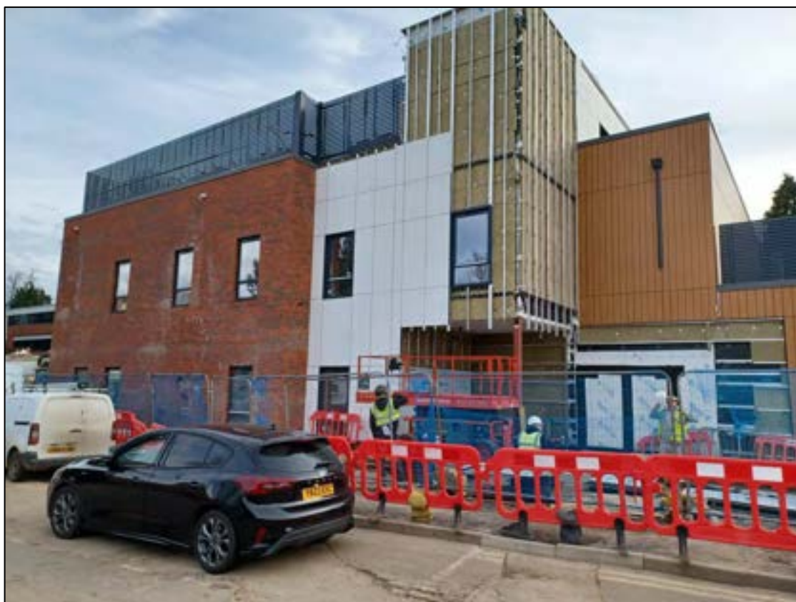
Photo 27 The new CDC Endoscopy building to the south-west of the Site
