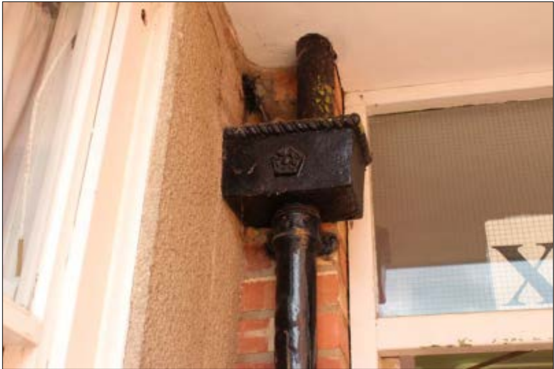
Photo 18 Cast iron rainwater goods with detail
