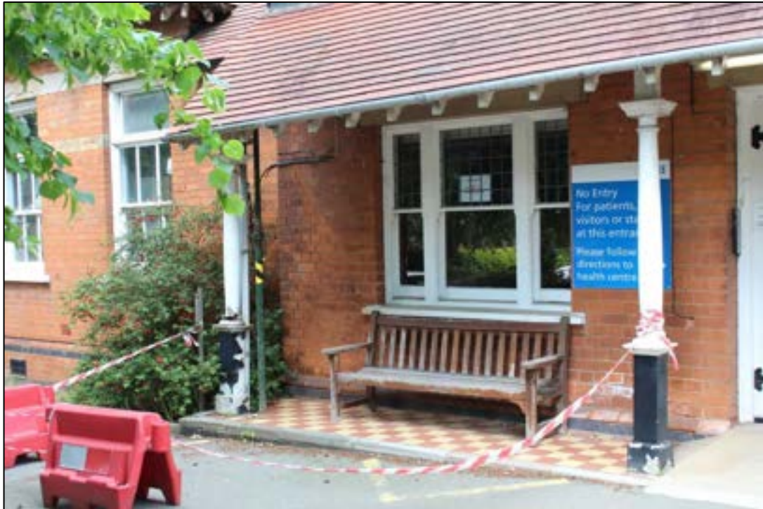
Photo 14 Tripartite sash adjacent to principle entrance (south-facing elevation)
