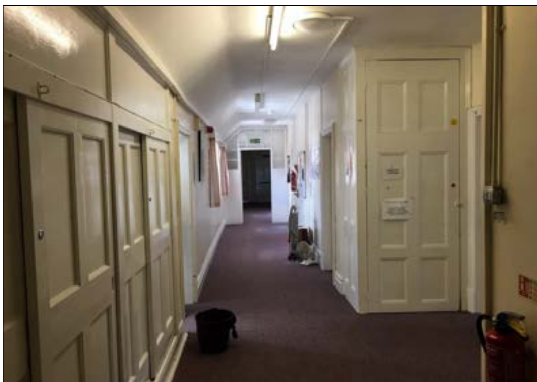
Photo 22 First floor central corridor
