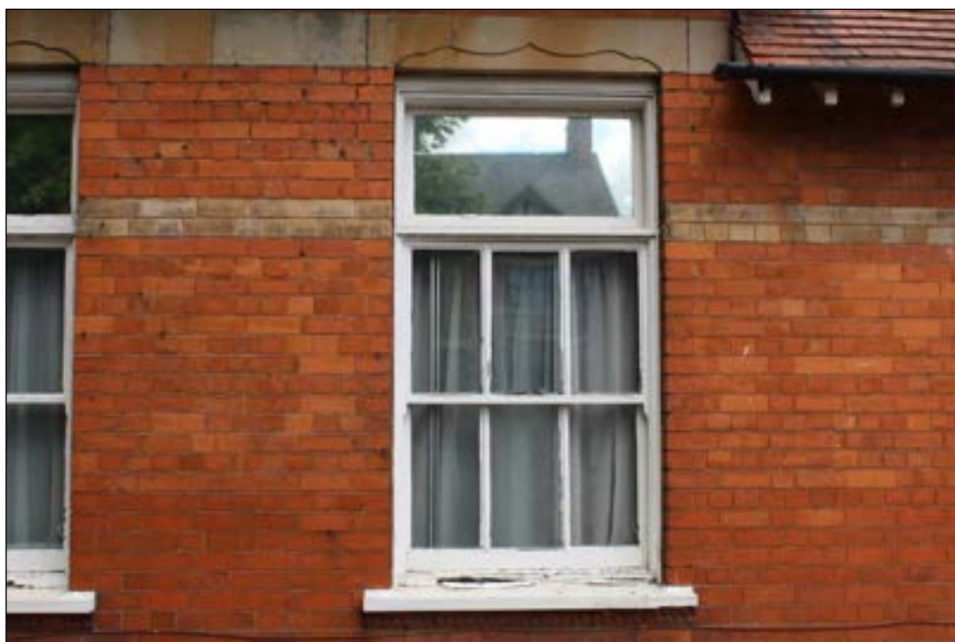
Photo 15 Sash window to the south facing elevation
