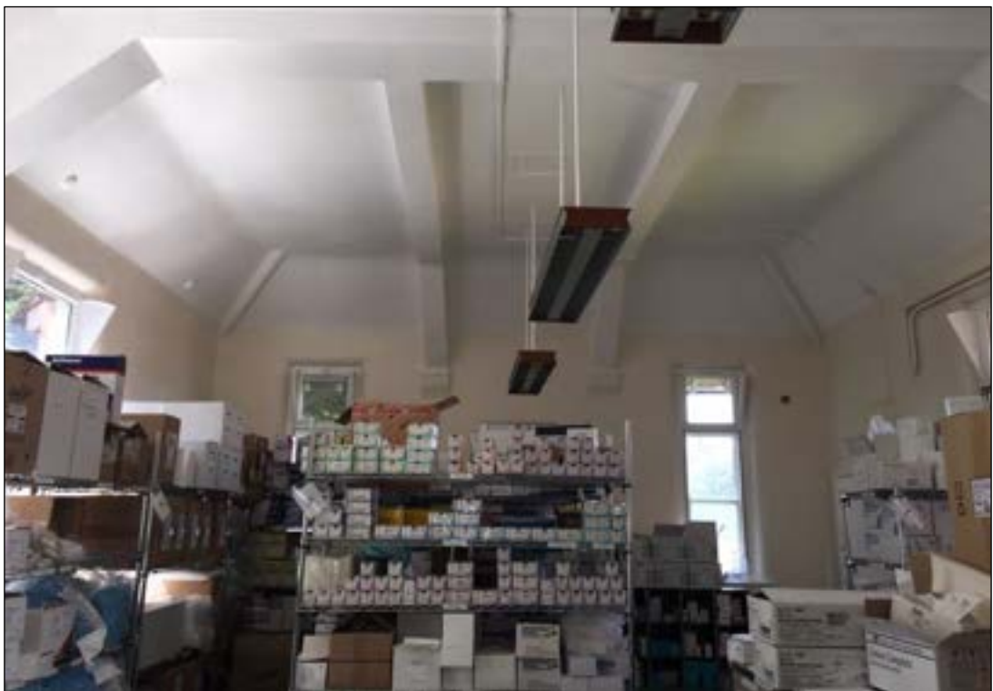
Photo 20 Original ward room to the left of the main entrance
