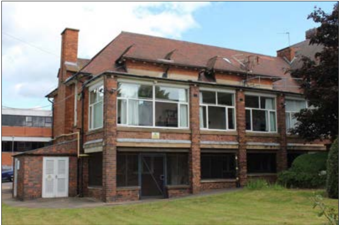
Photo 17 View of south-facing veranda windows on the north part of the west facing elevation, 1938 extension (now demolished)
