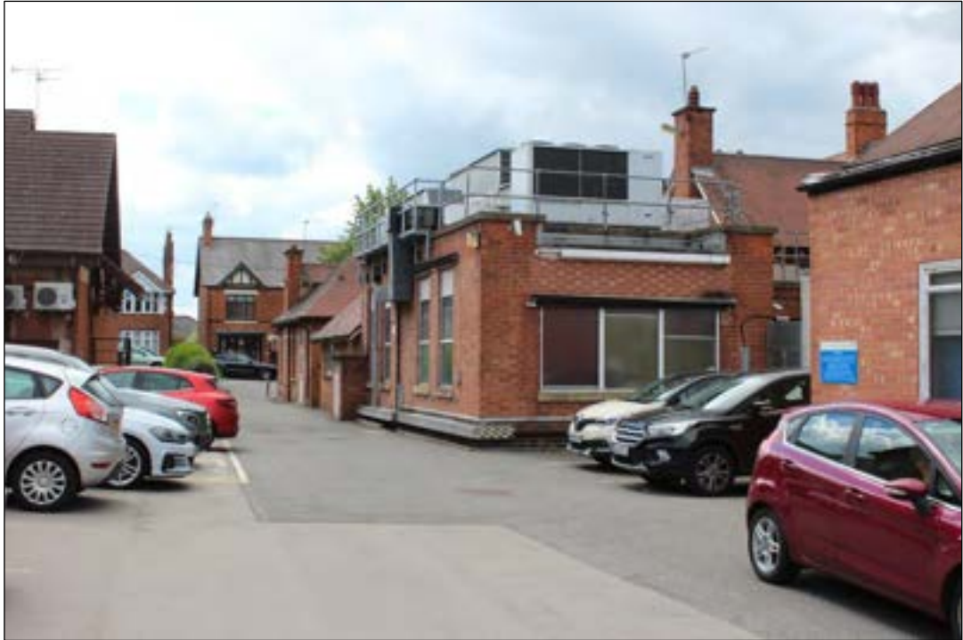
Photo 7 East-facing elevation of the Cottage Hospital viewed from car park showing the 1971 X-Ray Department, view to the south
