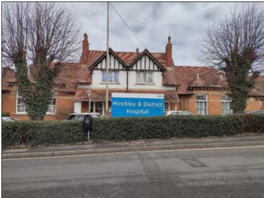
Photo 6 South-facing (principle) elevation of the Cottage Hospital
