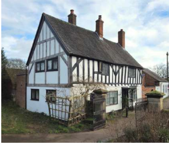
Archer Cottage Grade II Listed Entry No. 1361309
