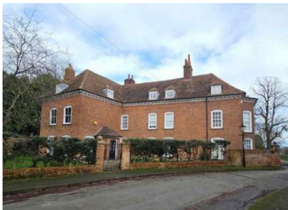
Burbage Hall Grade II Listed Entry No. 1074253
