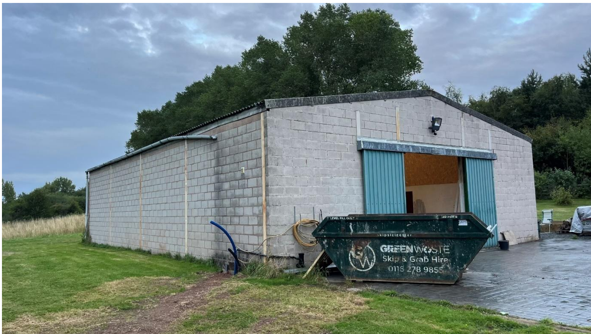
Photograph 1: The building taken from the south-west showing the breezeblock construction and large vehicle access doorway on the southern elevation.
