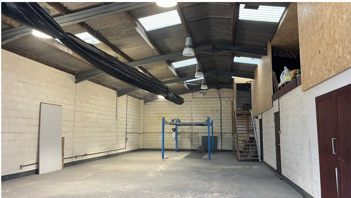
Photograph 3: The internal void of the building showing the steel frame with timber purlins and the workshops at ground floor level with storage area above.
