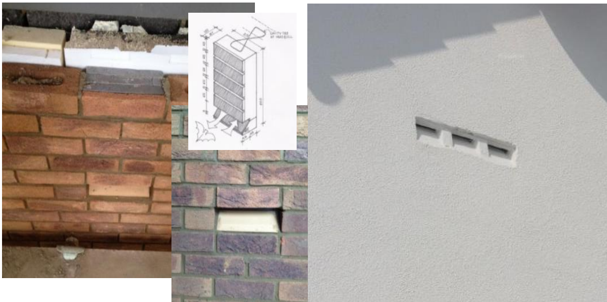
Figure 4: Examples of bat tubes fitted within the brickwork of an exterior wall, and within a white render.
