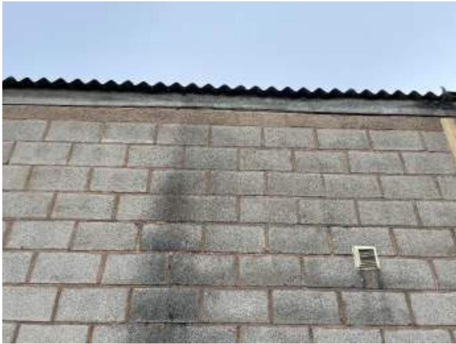
Figure 8: Damp staining on west wall
