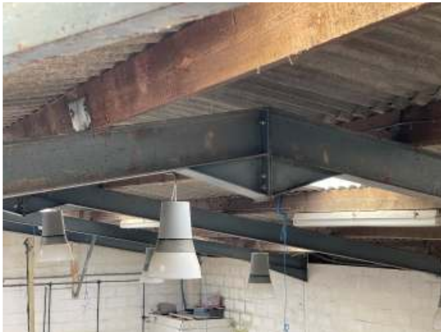
Figure 7: Portal frame ridge haunch
