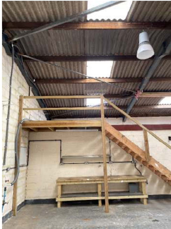
Figure 9: Roof bracing
