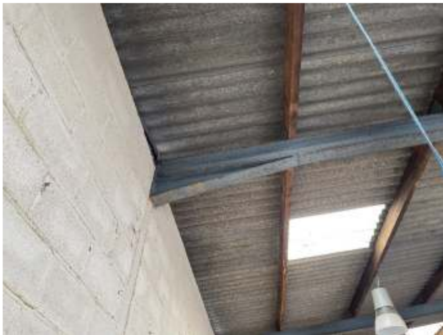
Figure 10: Timber purlins
