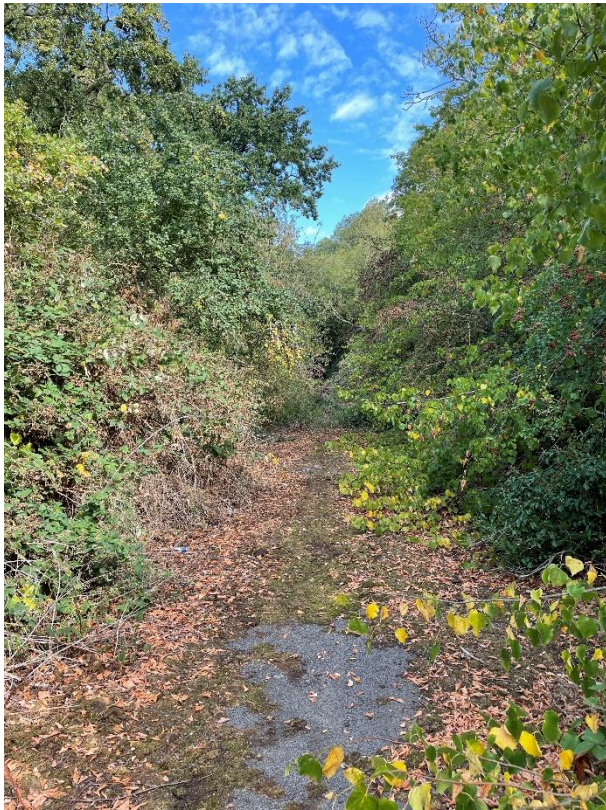
Figure 1.5 – Existing asphalt visible on Wolvey Road
