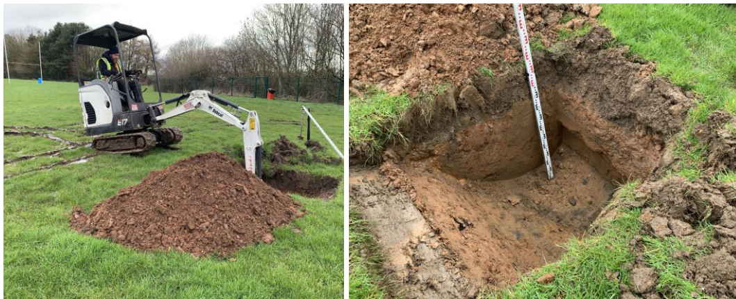
Trial Pit 3 – 150mm topsoil over compact clay loam subsoil, very wet surface
