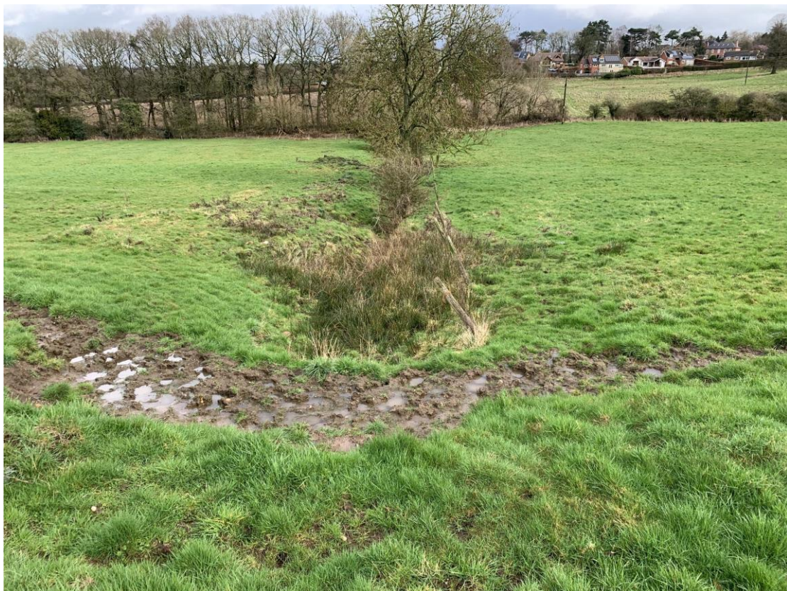
Potential existing outfall for playing fields, pasture land to the north. NB – an earthworks platform for stock gathering has been constructed over the point where an outfall from the playing field system may have run.
