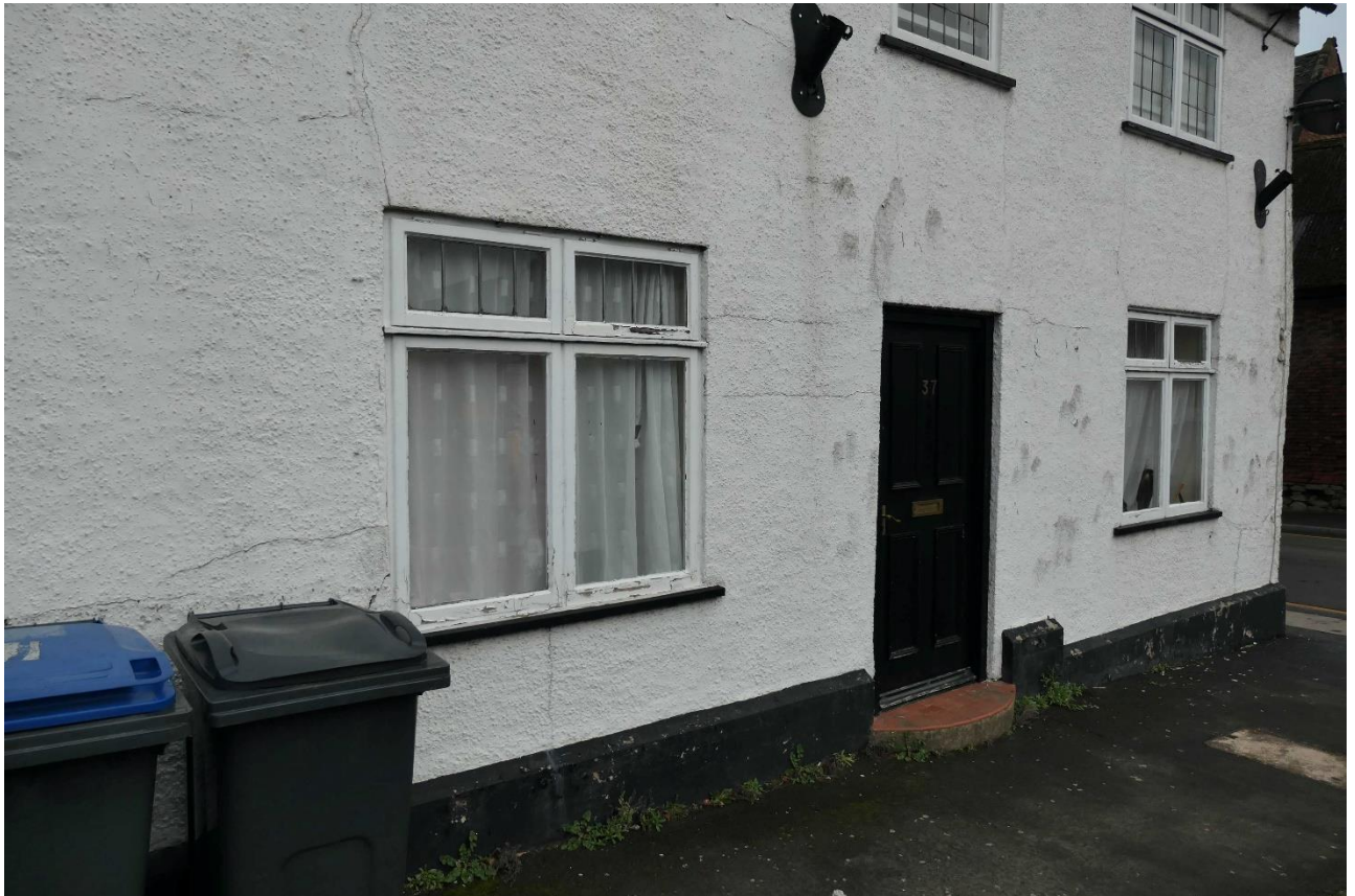
Photo 6: A detail of 37 High Street.
