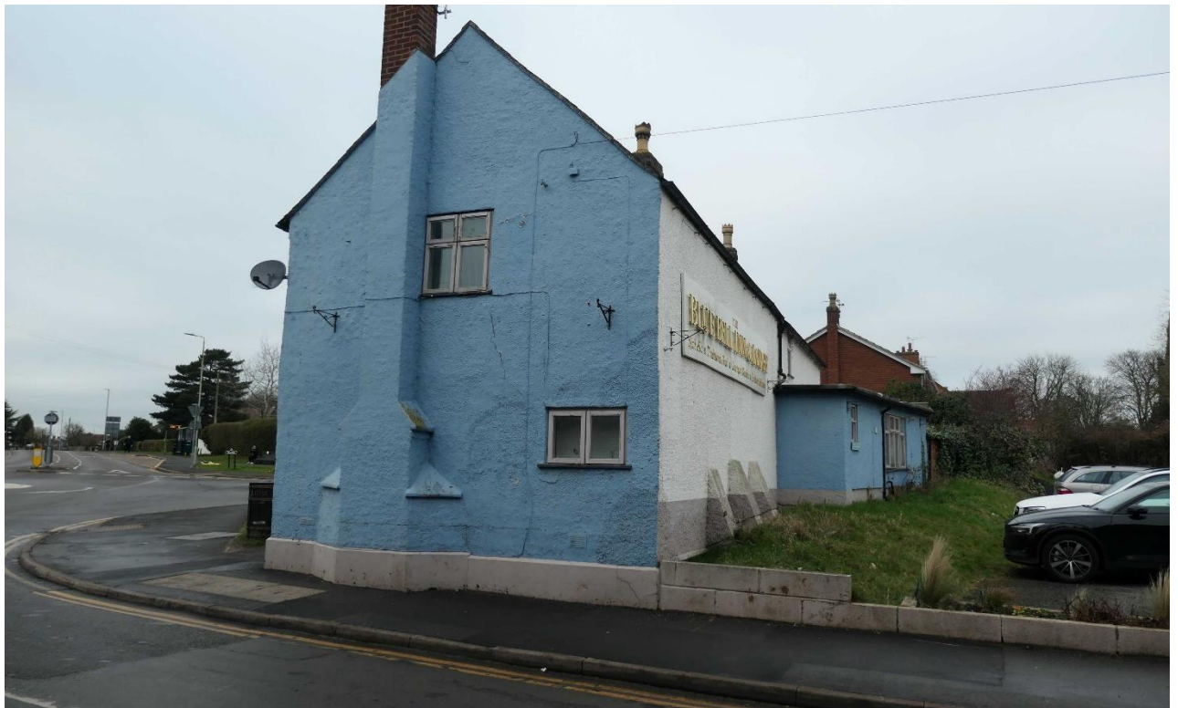
Photo 3: The south gable of 37 High Street.
