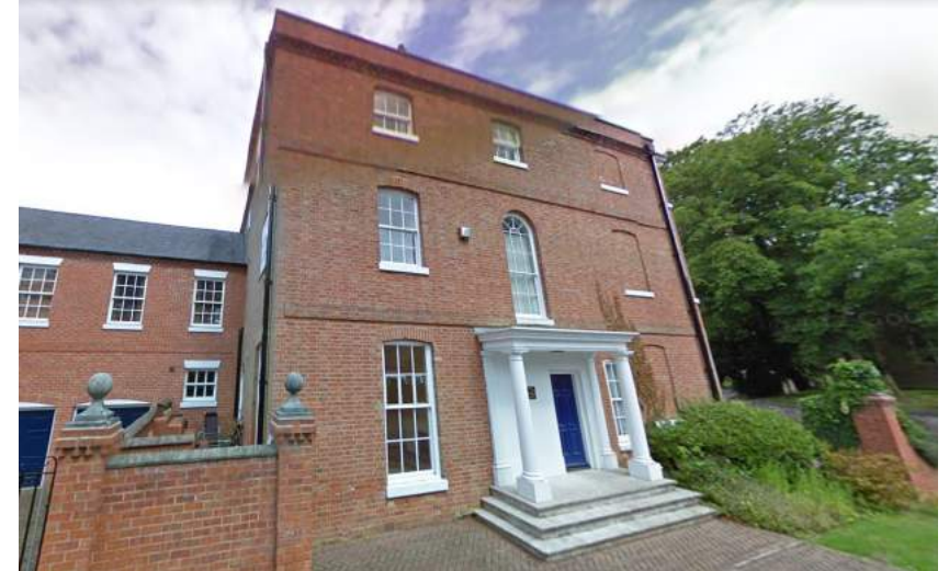
Brick Banding, Eaves Detail and Recessed Brick Details
