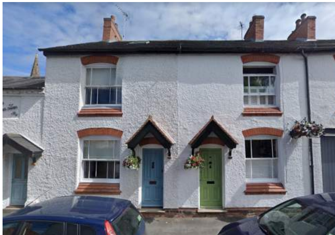
Brick Lintel and Sill Details
