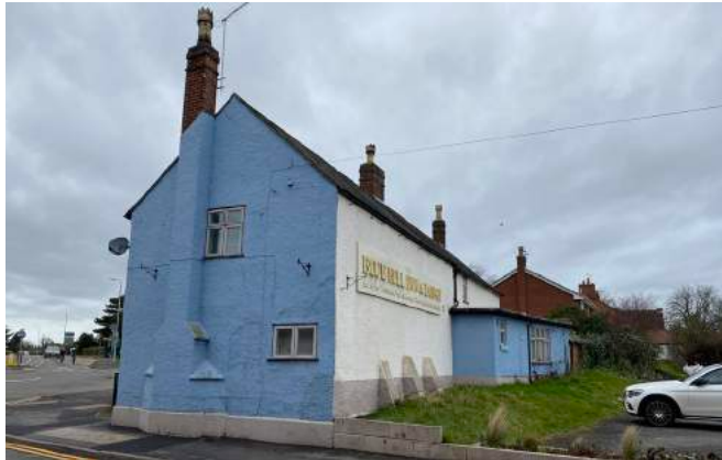
View 2: Looking North-West from High Street
