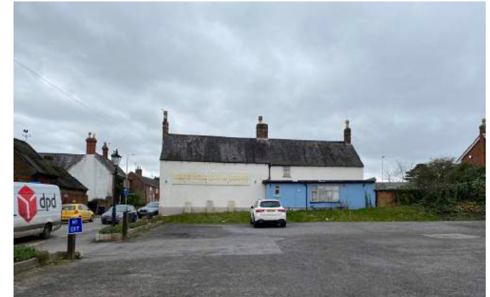
View 3: Looking West from the Car Park
