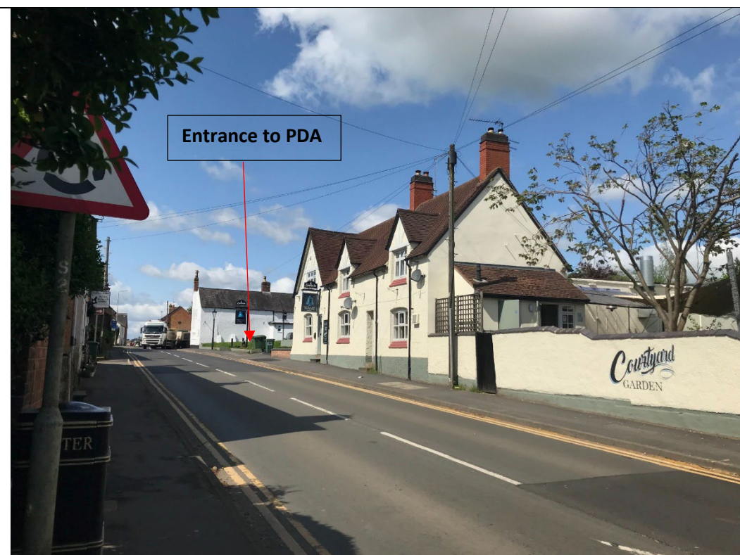
Plate 1: The Blue Bell Inn viewed from High Street. Entrance to PDA visible
