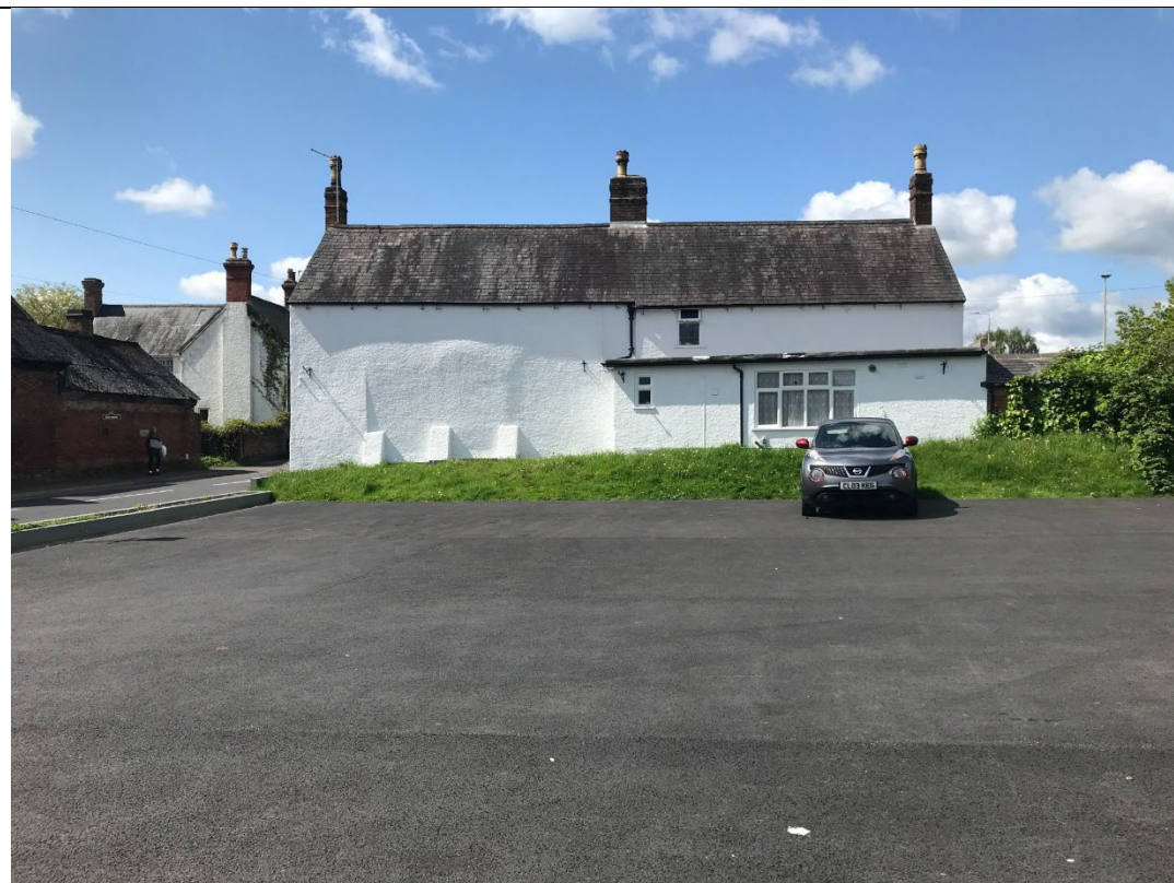
Plate 5: Facing west across the southern part of the PDA. The rear of No 37 High Street and No 2a Main Street are visible in the centre of this image
