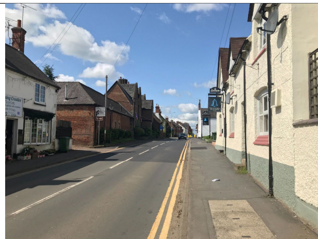
Plate 2: Facing west along High Street. Blue Bell Inn on right hand side of image. Entrance to PDA visible
