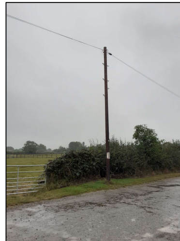
Photo 4: Overhead electricity cables which run parallel to the access track in the north-west.
