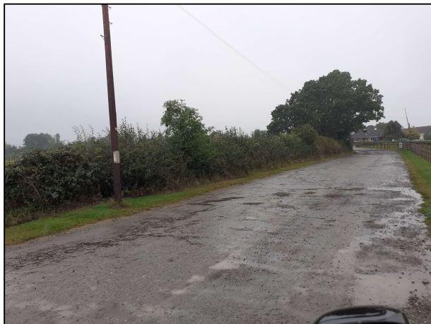
Photo 3: View looking south-east across the access track in the north-west.
