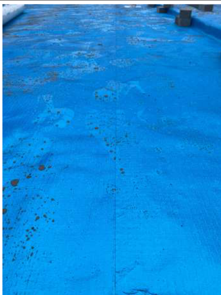
An overview of a welded lap joint.
