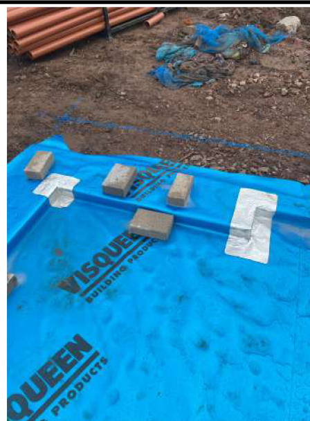
Sealed corner and perimeter details.
