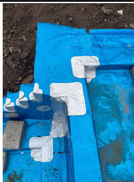
Visqueen GR SAM was used to seal corner details.
