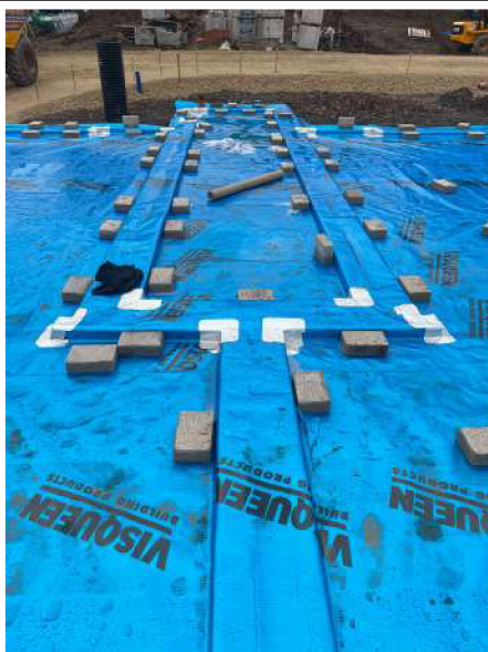
An overview of internal walls and sealed corner details.
