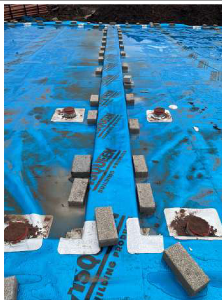
An overview of an internal wall and sealed corner and pipe penetrations.
