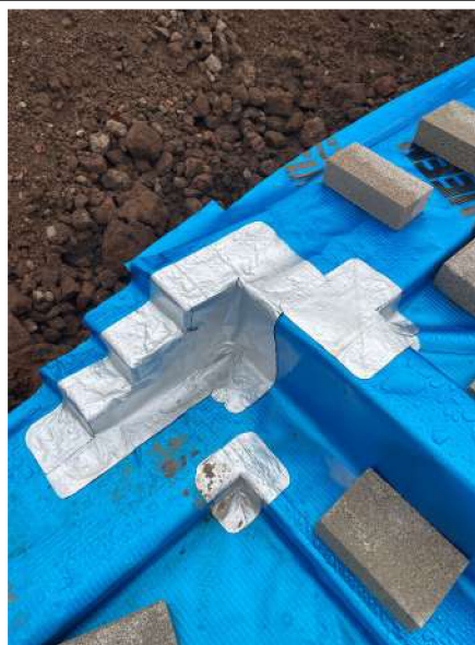
All corner details were sealed with Visqueen GR SAM.
