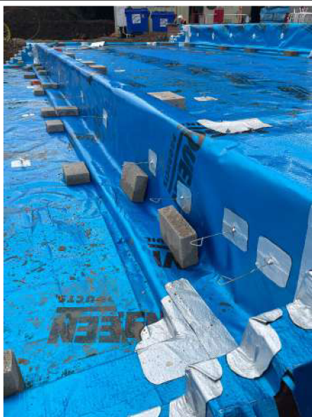
Visqueen Standard Gas Barrier has been installed tightly across two plots.
