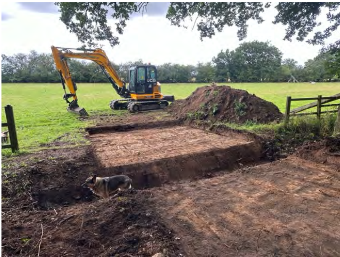
Plate 4: Road access fully stripped looking north.
