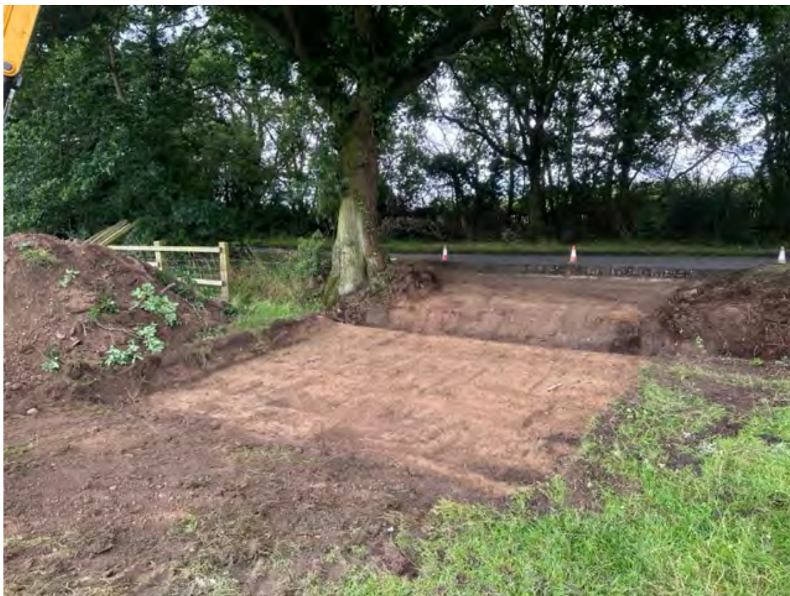
Plate 3: Road access fully stripped looking south-east.
