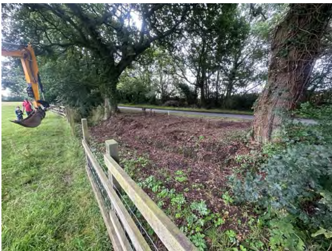
Plate 2: Road access prior to stripping looking south-east.
