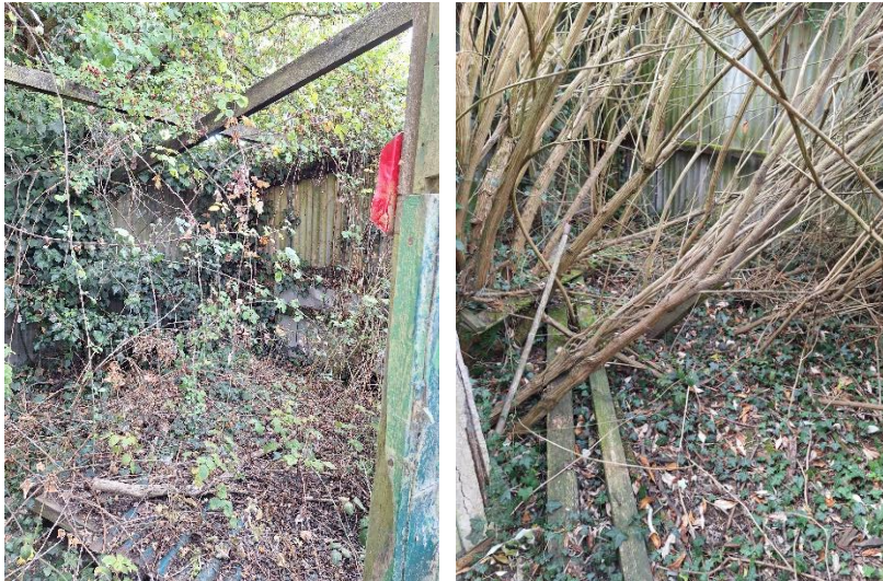
Photographs 10&11: vegetation growing inside the structure.
