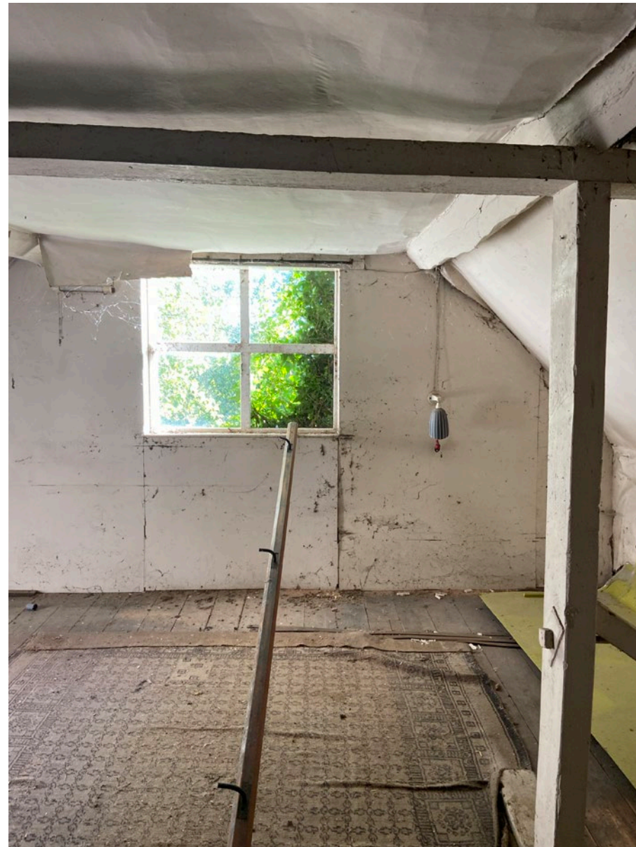
VIEW OF AN ATTIC ROOM
