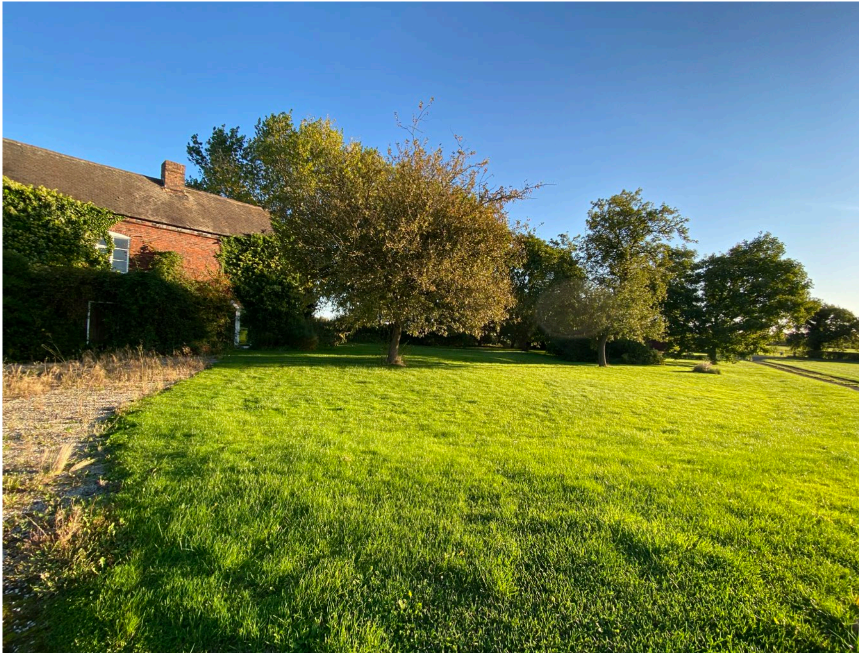
VIEW OF THE FRONT OF FROG HALL FARMHOUSE LOOKING NORTH EAST
