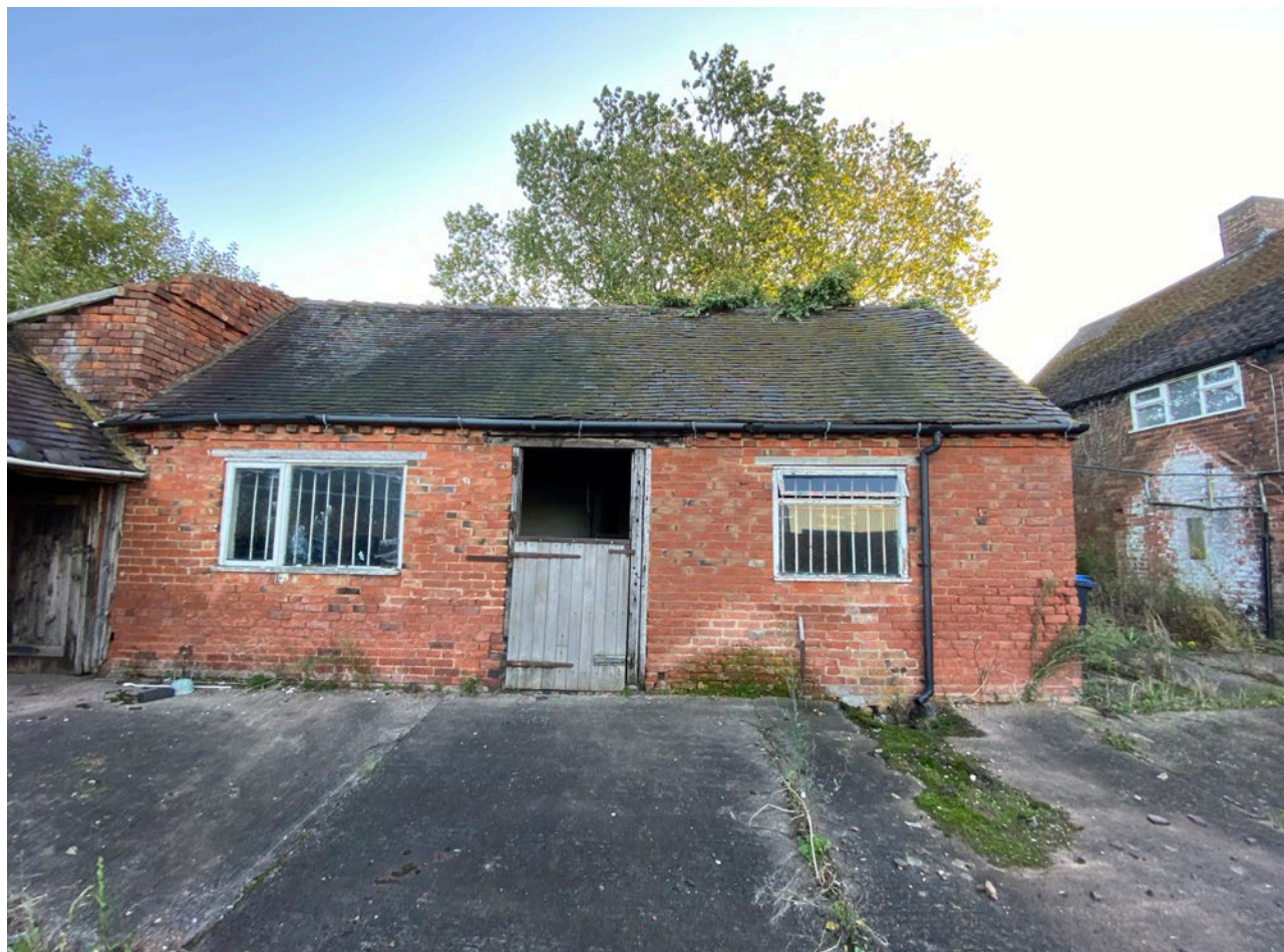
VIEW OF THE FRONT OF ONE OF THE OUTBUILDINGS LOOKING EAST
