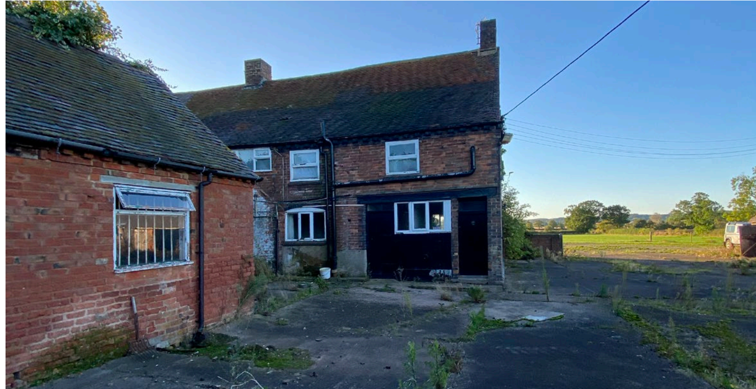
VIEW OF FROG HALL FARMHOUSE LOOKING SOUTH
