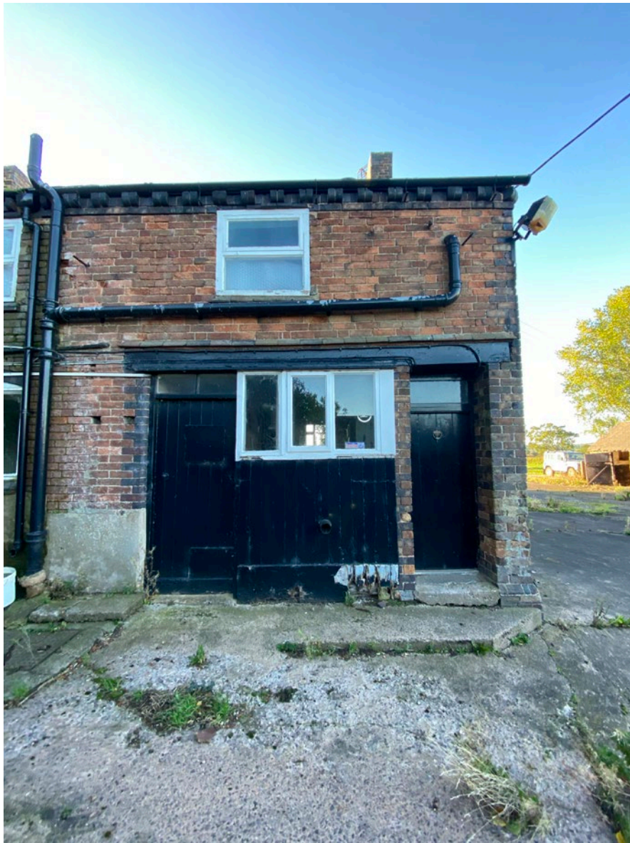
VIEW OF THE REAR OF FROG HALL FARMHOUSE LOOKING SOUTH
