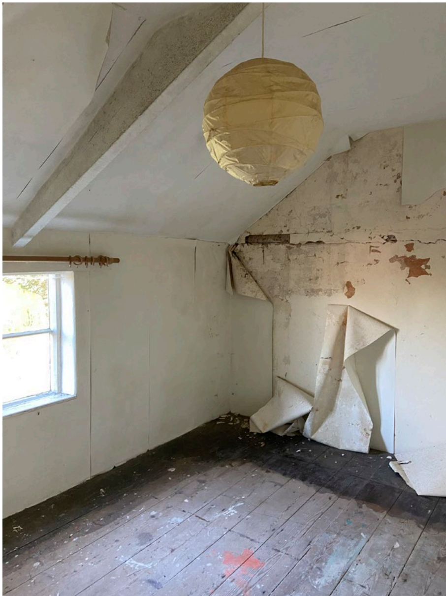
VIEW OF A FIRST FLOOR ROOM
