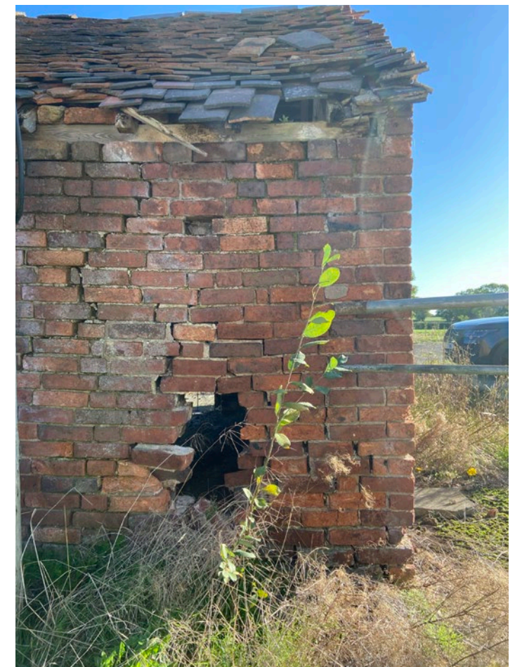
VIEW OF THE REAR OF ONE OF THE OUTBUILDINGS LOOKING EAST
