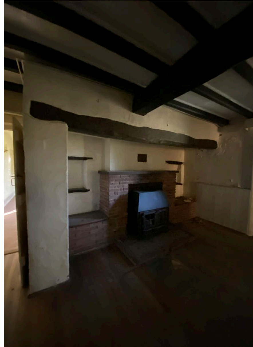
VIEW OF A GROUND FLOOR ROOM
