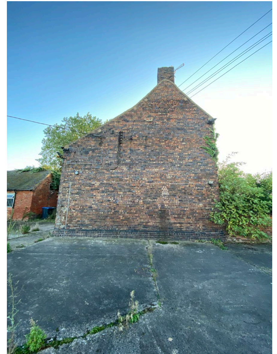
VIEW OF THE GABLE END OF FROG HALL FARMHOUSE LOOKING EAST
