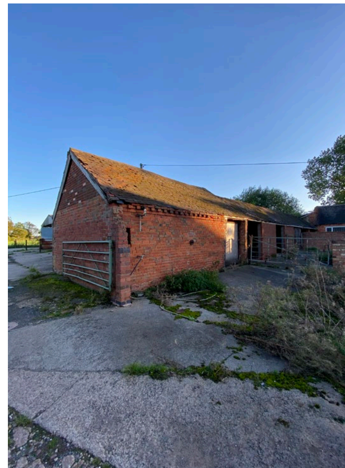
VIEW OF THE FRONT OF ONE OF THE OUTBUILDINGS LOOKING NORTH WEST
