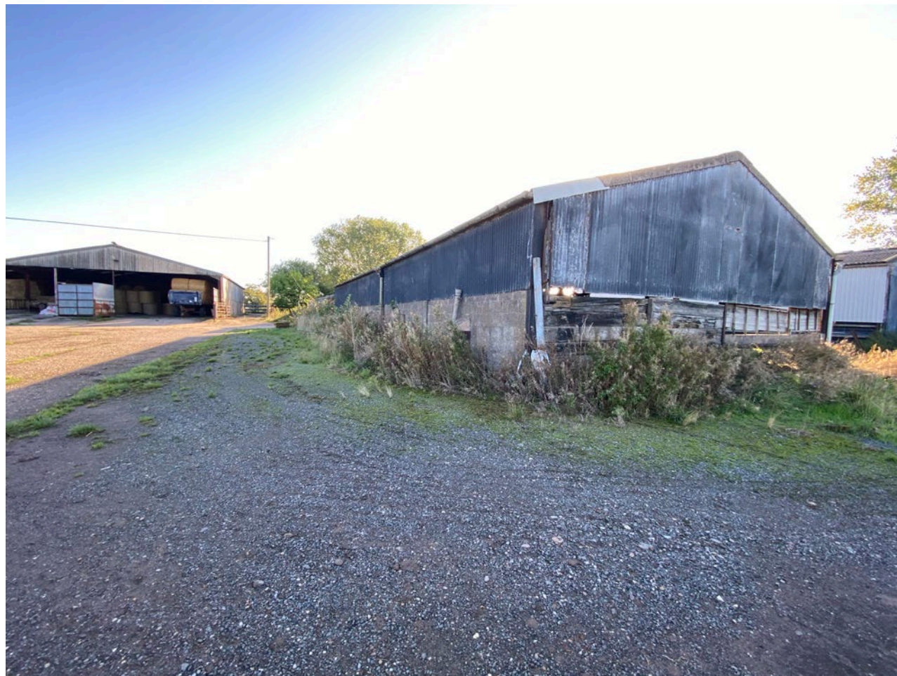
VIEW OF THE FRONT OF ONE OF THE AGRICULTURAL BARNs LOOKING SOUTH EAST
