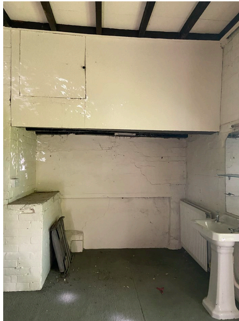
VIEW OF A FIRST FLOOR BEDROOM
