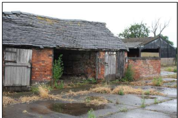
Figure 19. Hard Standing around Farm Buildings
