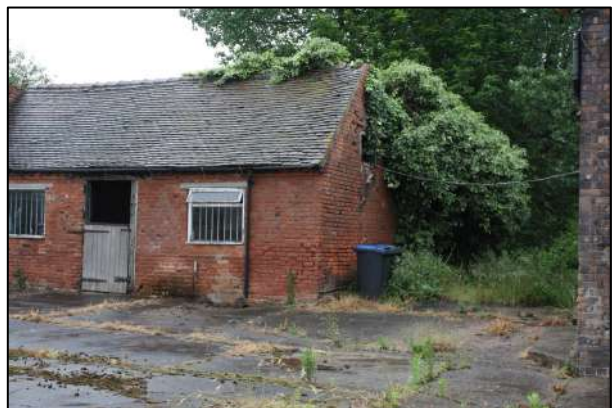
Figure 17. Hard Standing around Farm Buildings
