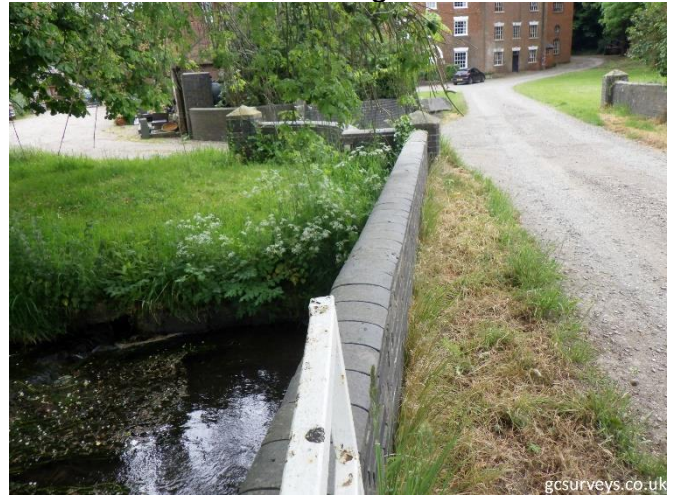
Downstream Face, looking west
