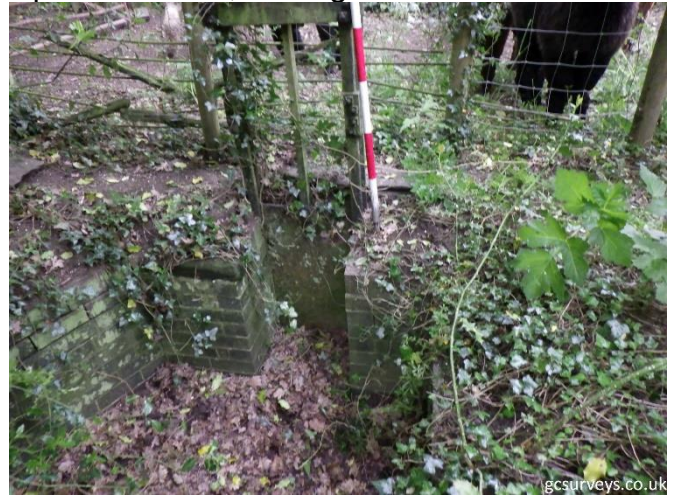
Upstream Face, looking Downstream
