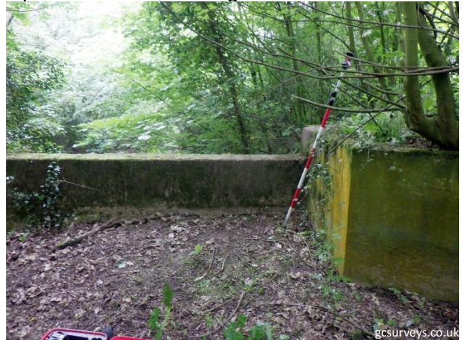
Upstream Face, looking Downstream
