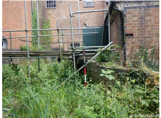
Upstream Face, looking Downstream
