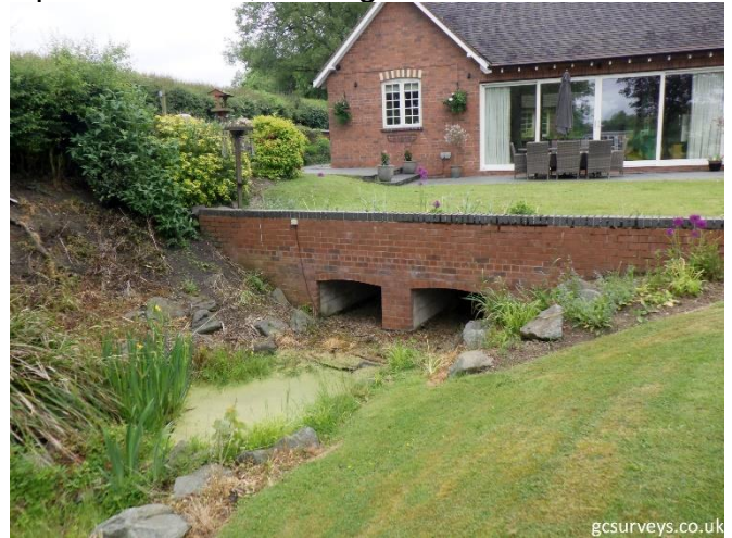
Upstream Face, looking Downstream
