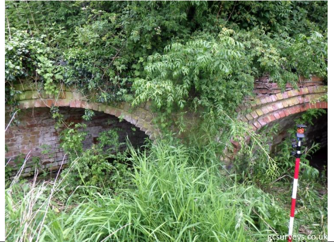
Upstream Face, looking Downstream
