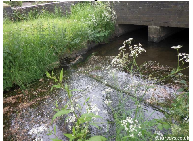
Upstream Face, looking downstream
