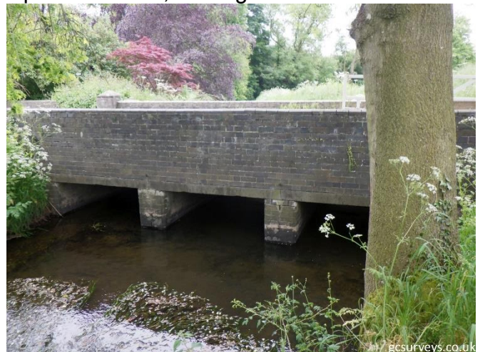
Upstream Face, looking downstream
