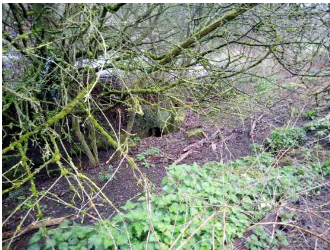
Plate 8: view south-west of stream and culvert
