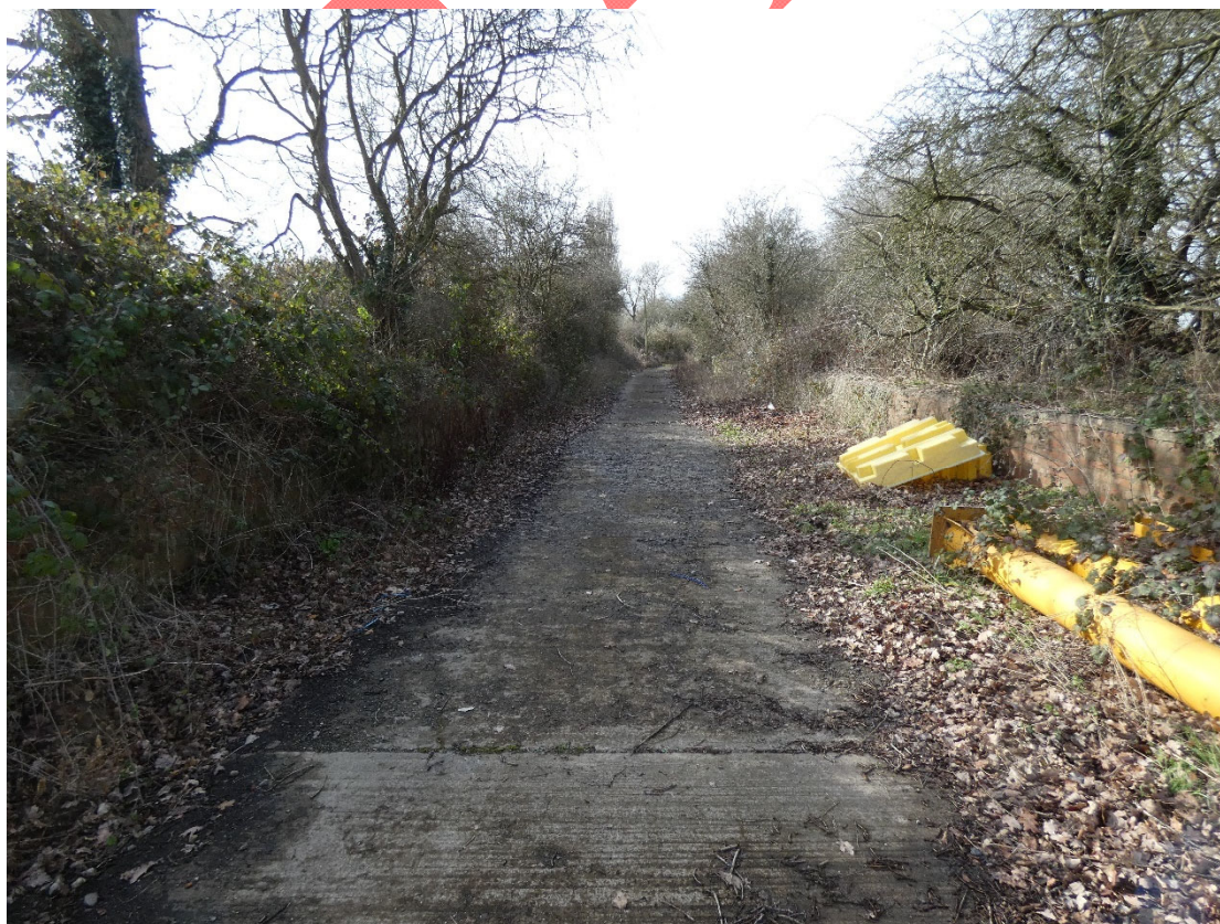
Figure 20: The concrete path extending into the southern section (looking south).
