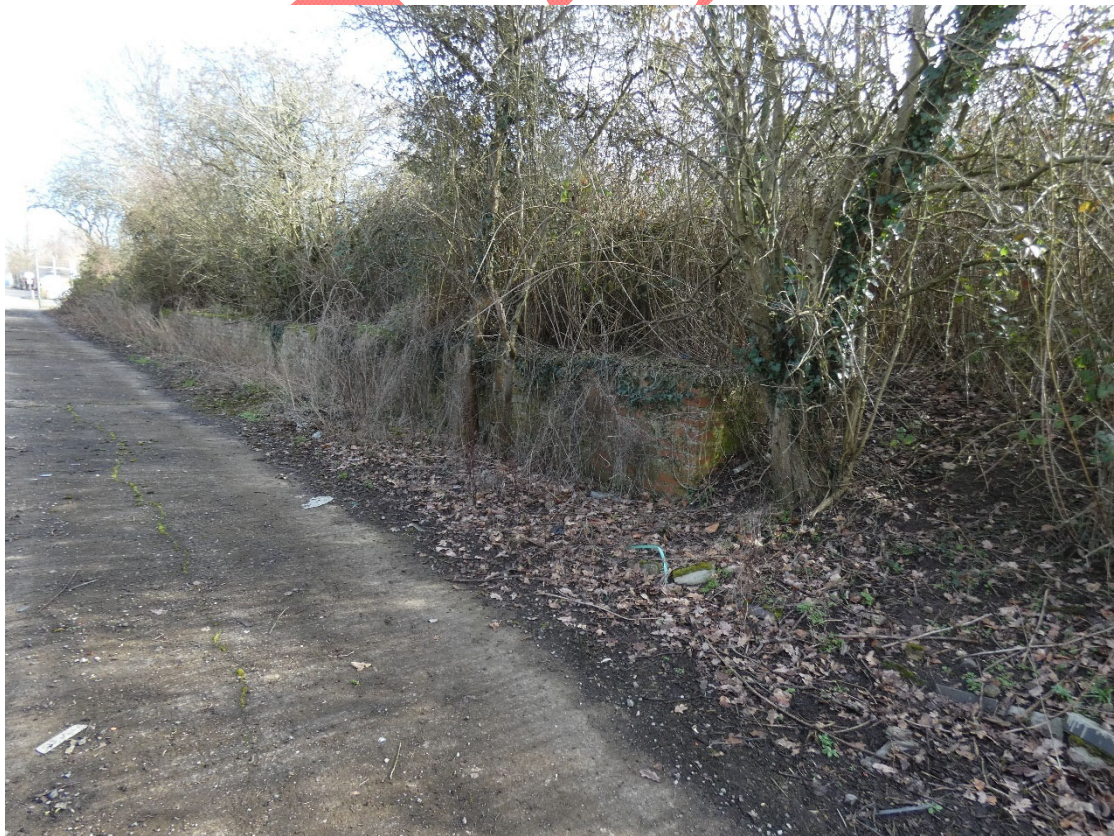
Figure 23: The overgrown eastern wall flanking the path (looking north-east).
