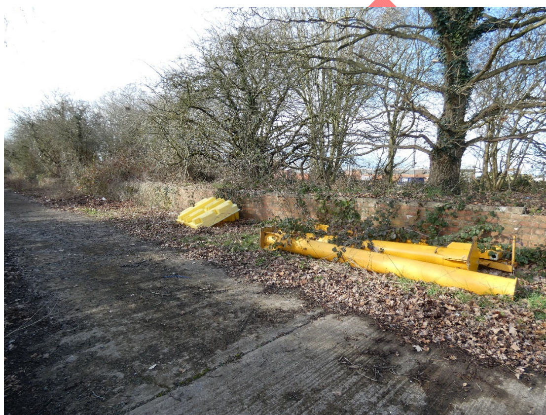
Figure 24: The western wall flanking path (looking south-west).
