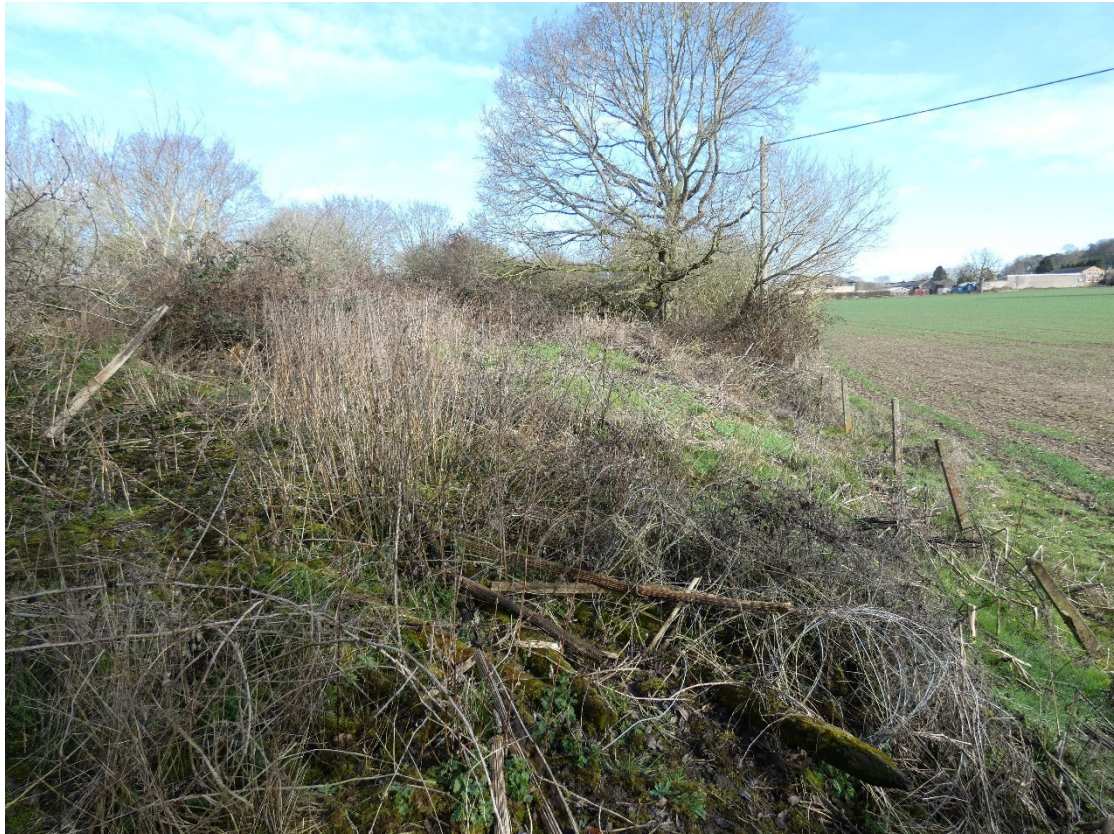
Figure 22: The eastern boundary in the southern section of the site showing the large embankment found to the east of the concrete path (looking north).
