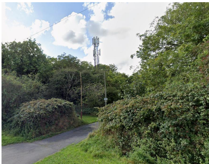
Figure 3. View of the existing site from Newtown Linford Lane (Source: Google Maps).
