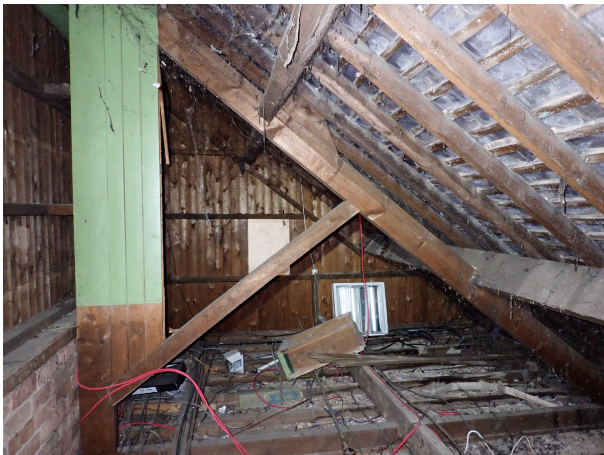
10 – A small roof void to the rear has no lining, and is filled with dusty cobwebs.
