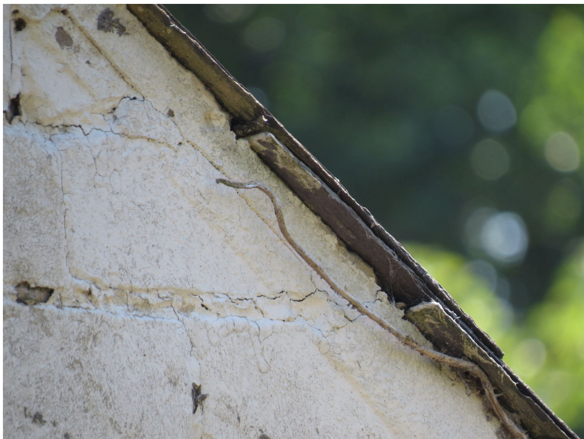
8 – End tiles at the verges are sealed with cement.
