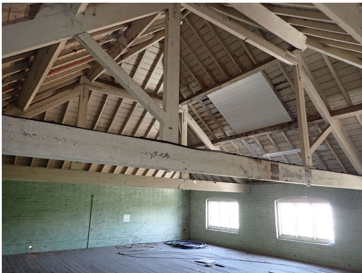
9 – The main section the roof has no enclosed roof void.
