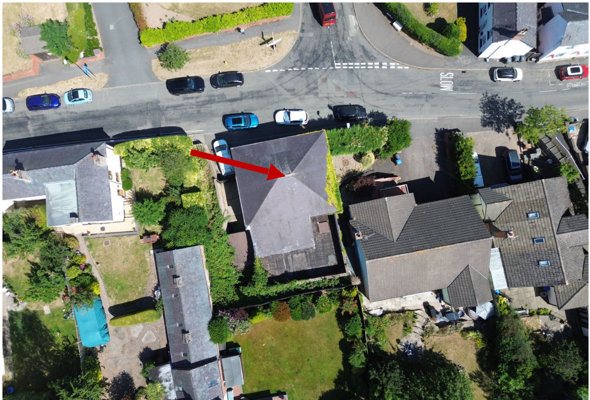
1.6b – 23 Newbold Road – aerial photograph.
