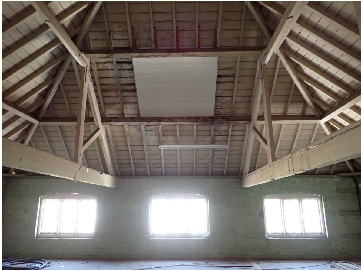
3.2a – The roof void.
