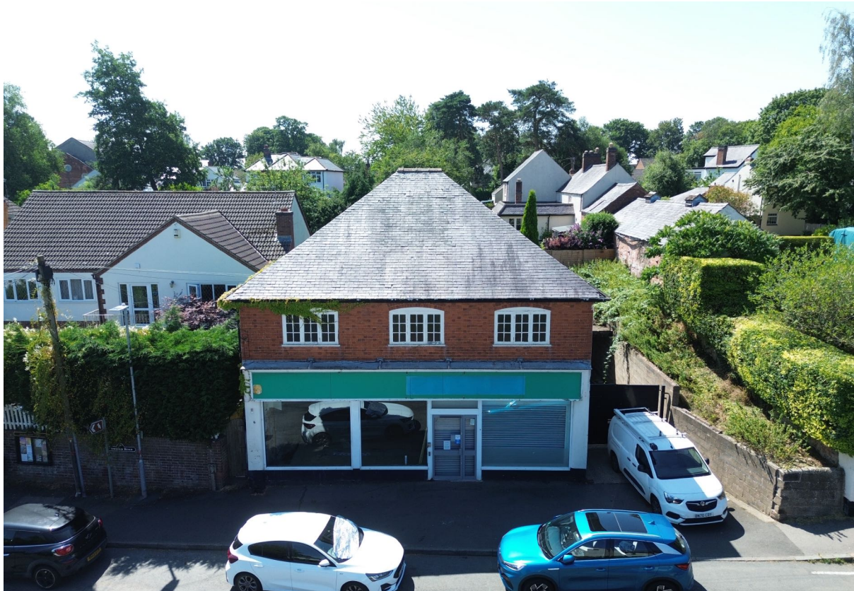
1 – The front of the building.
