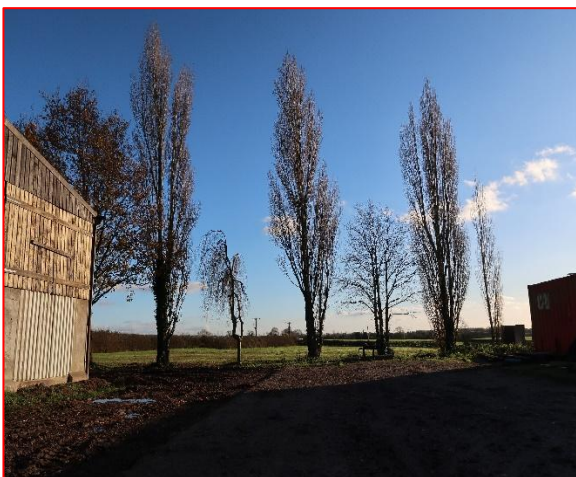
View of building & Poplar trees to boundary
