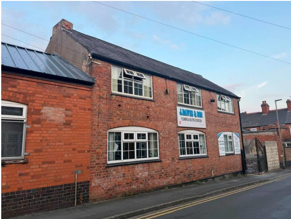
North and west elevations of western building
