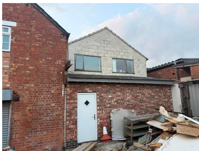
South elevation of eastern building and extension
