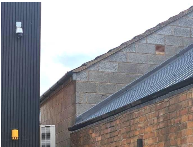
North and east elevations of eastern building
