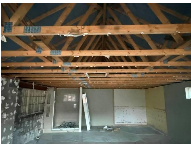
Upper floor of eastern building
